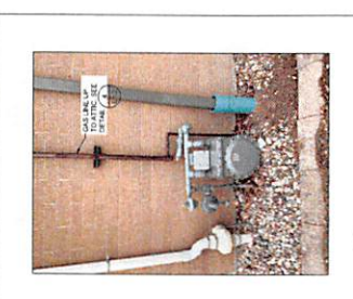
1 EXISTING GENERATOR GAS PIPING E1.2 NTS
