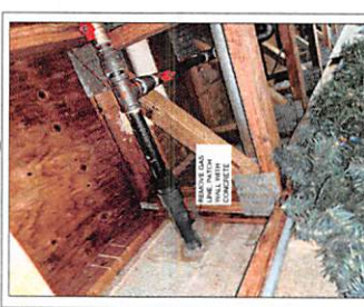
1 EXISTING GENERATOR GAS PIPING E1.2 NTS
