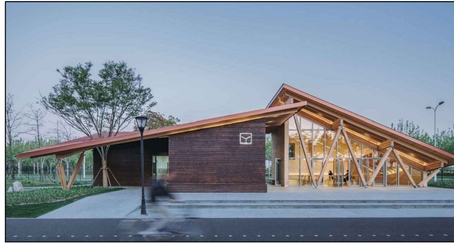
Combined Restrooms and Interior Space
