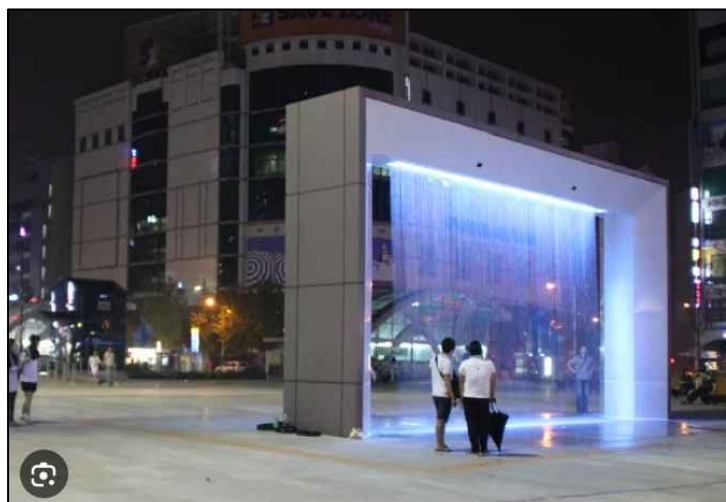
Water Curtain - South Korea
