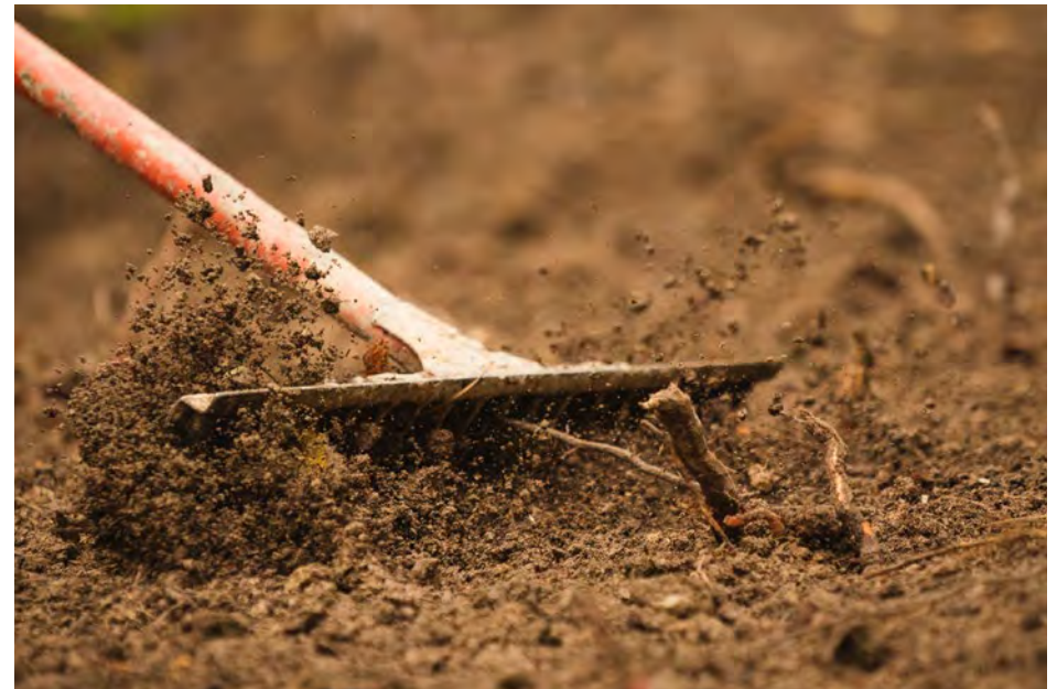
Trail construction employs a host of advanced tools, but sometimes the job simply calls for the time-tested rake.
