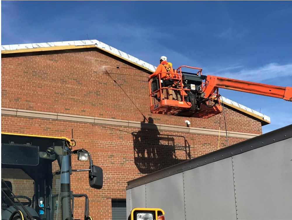
Pump station face brick washing.
