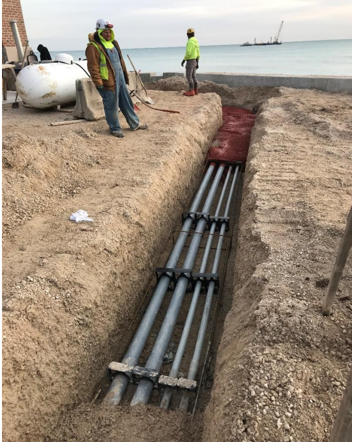
Electrical ductbank concrete placement.
