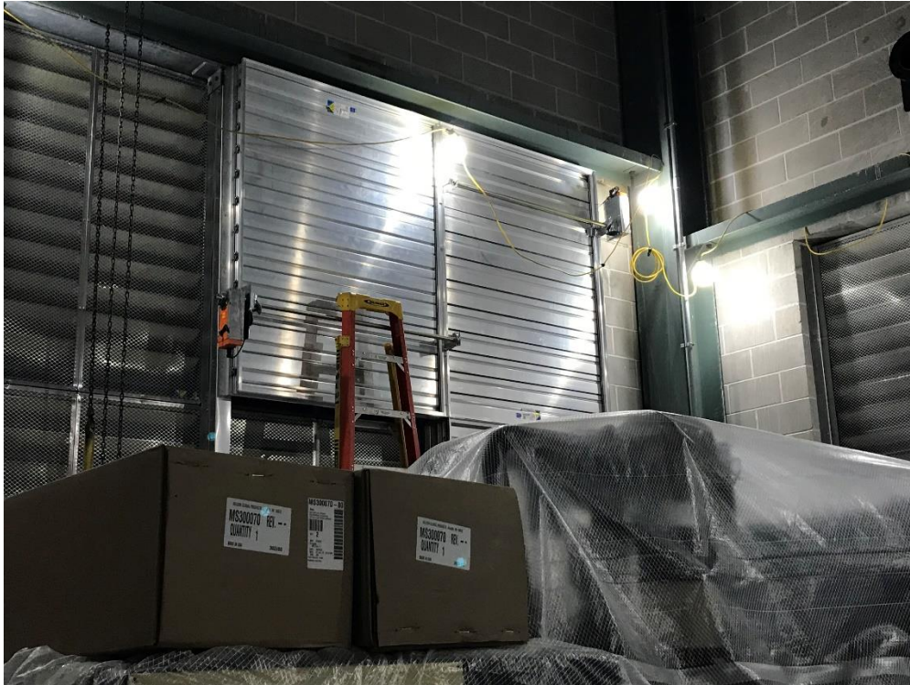
Louvers and dampers installed in generator room.
