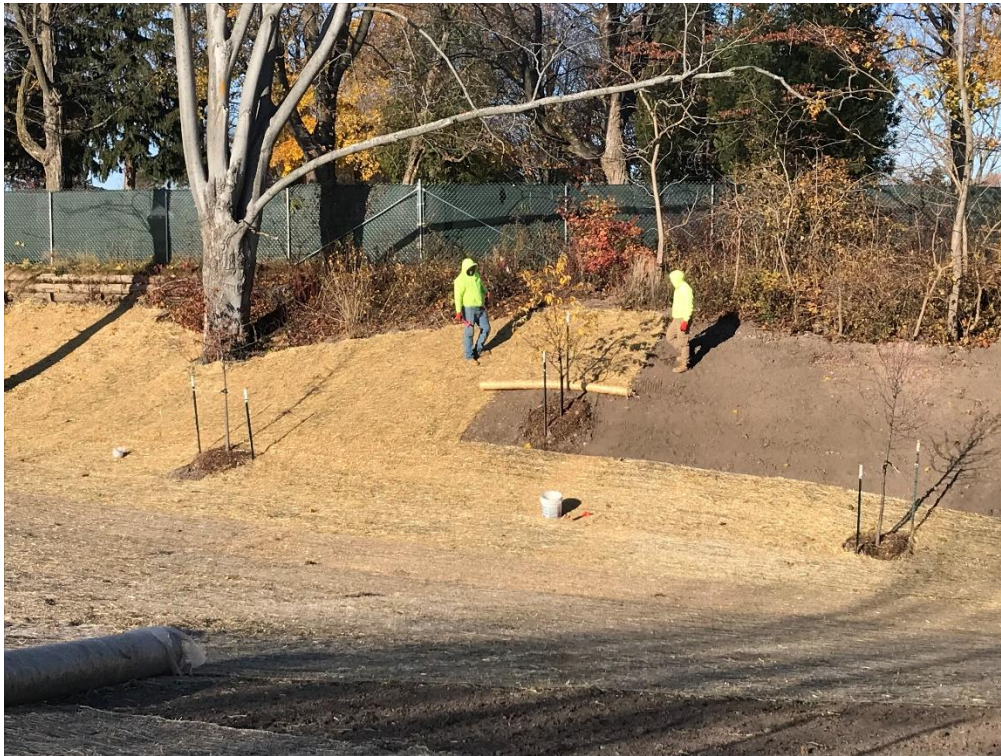
Seed and erosion control mat installed in ravine.
