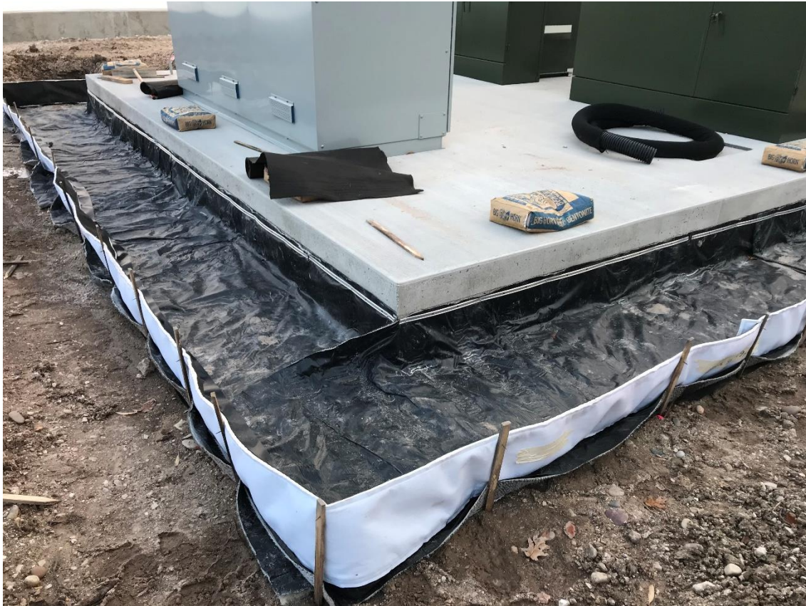
Oil containment installation at transformer pad.
