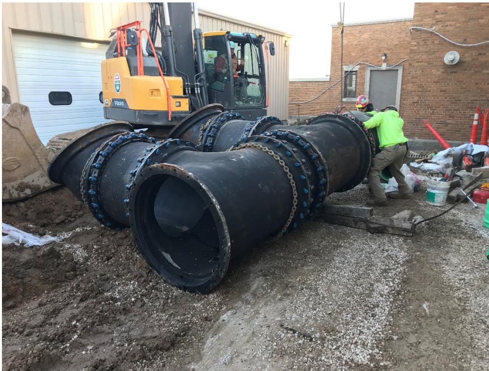
36" RW pipe assembled for tie-in.
