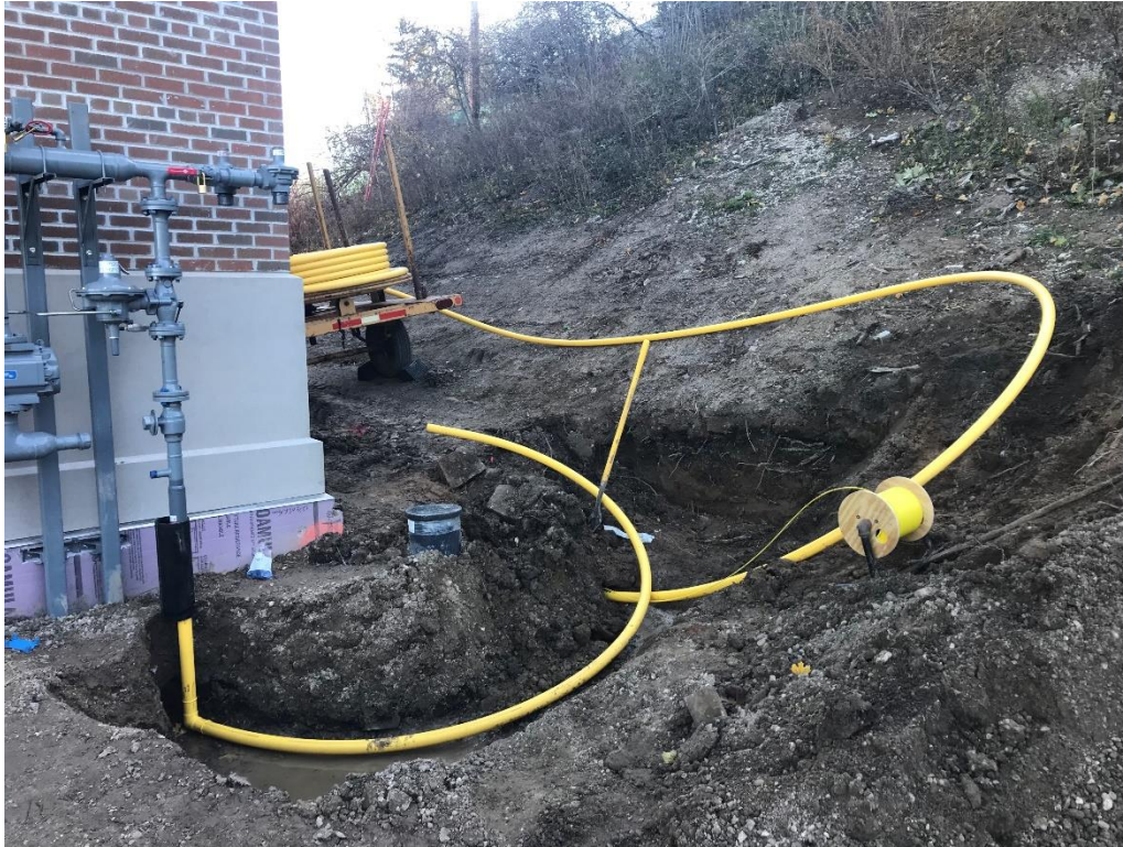
Gas pipe, meter and valve assembly installed at pump station.
