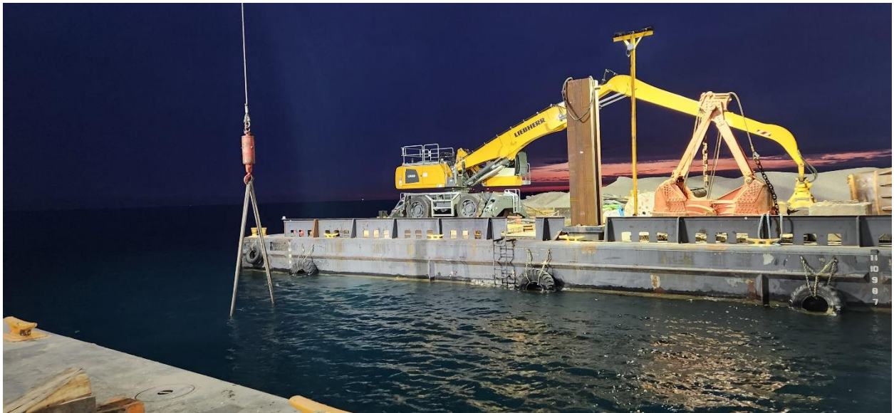
Kokosing prepares to place bedding stone at installed intake pipe.
