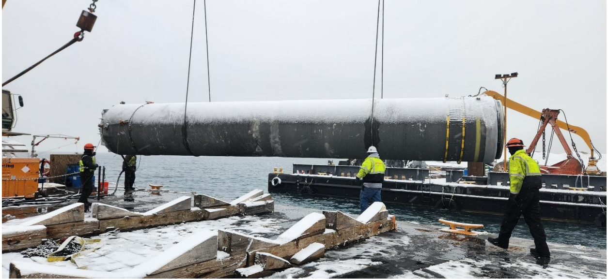
Kokosing prepares to install intake pipe.
