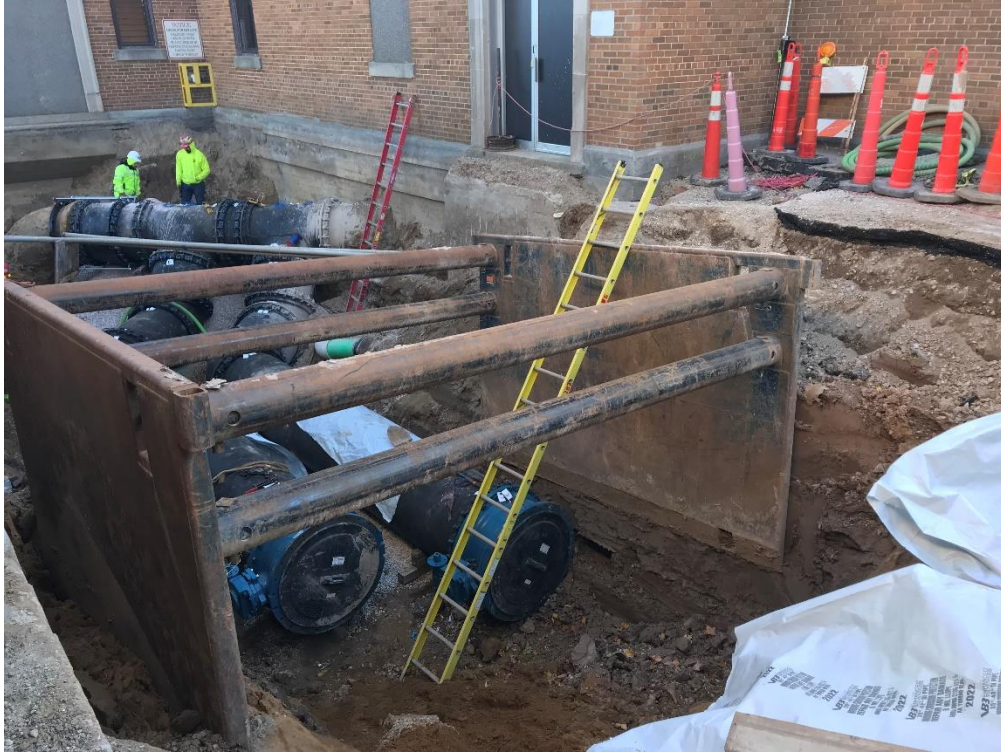
36" RW pipe installed at tie-in location.
