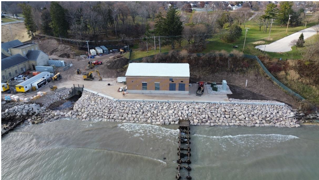
Completed revetment stone placement.
