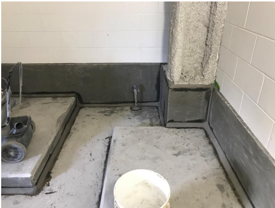
Resinous floor installation in chemical room.
