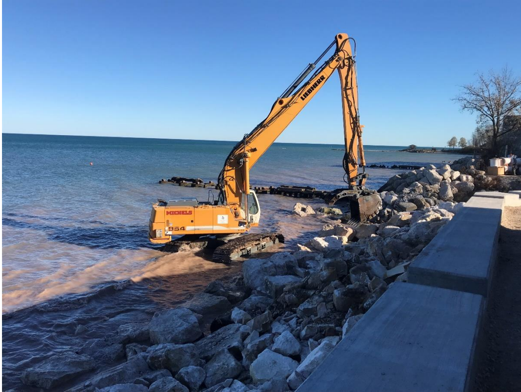
Michels installs revetment stone.
