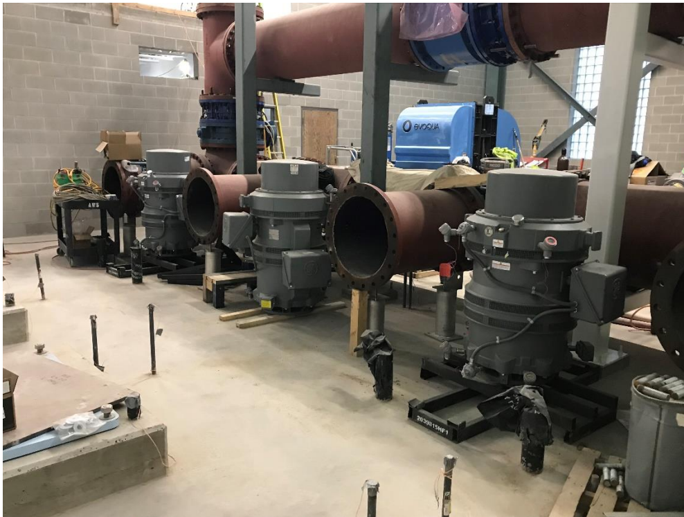
Pump motors located in pump room.
