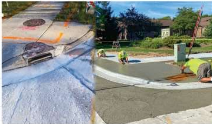
ADA-compliant ramp installation
