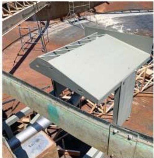
New scum box installed on Primary Clarifier #4
