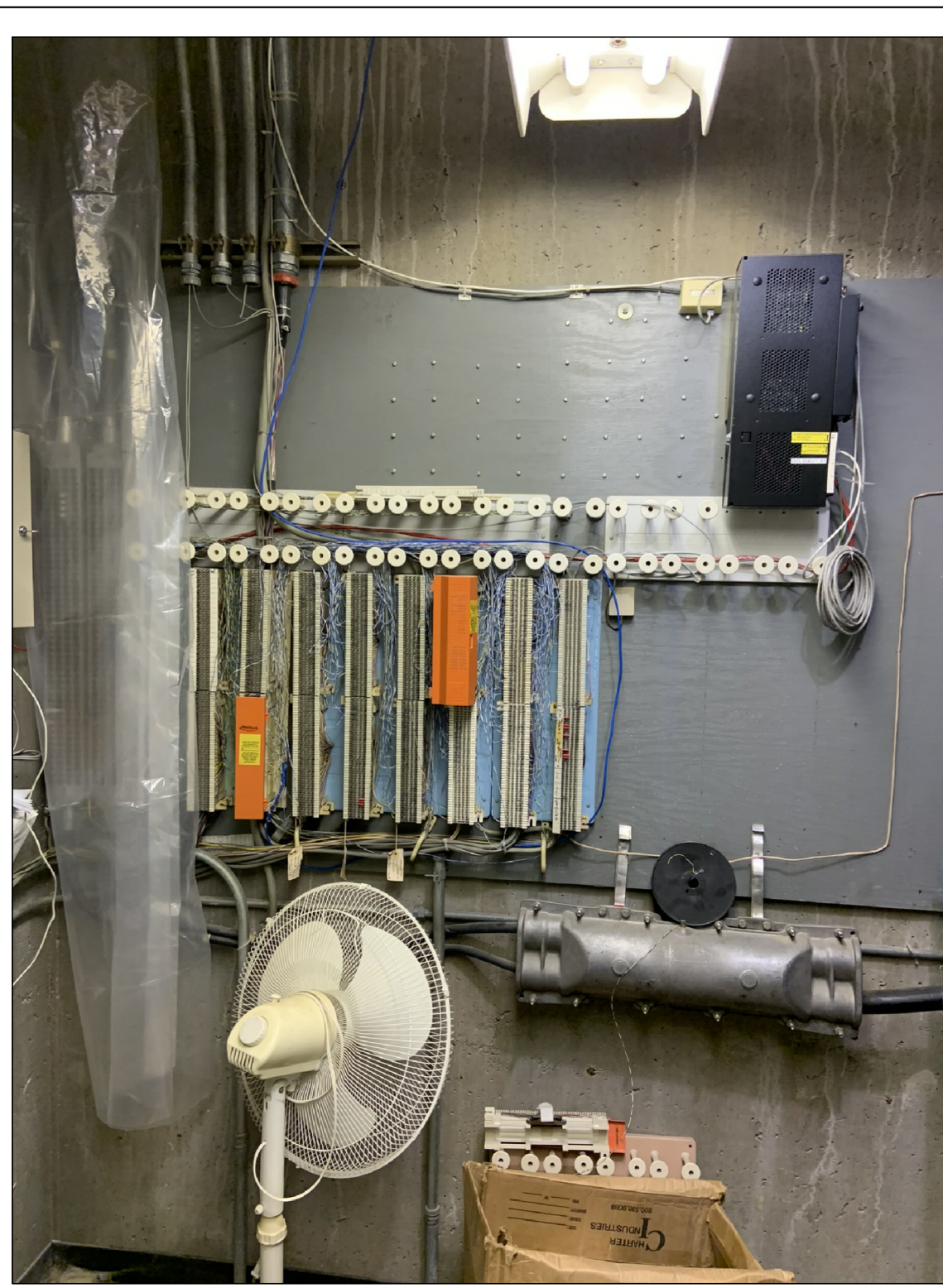
2 E1.0D EXISTING TELEPHONE TERMINATION BOARD NTS
