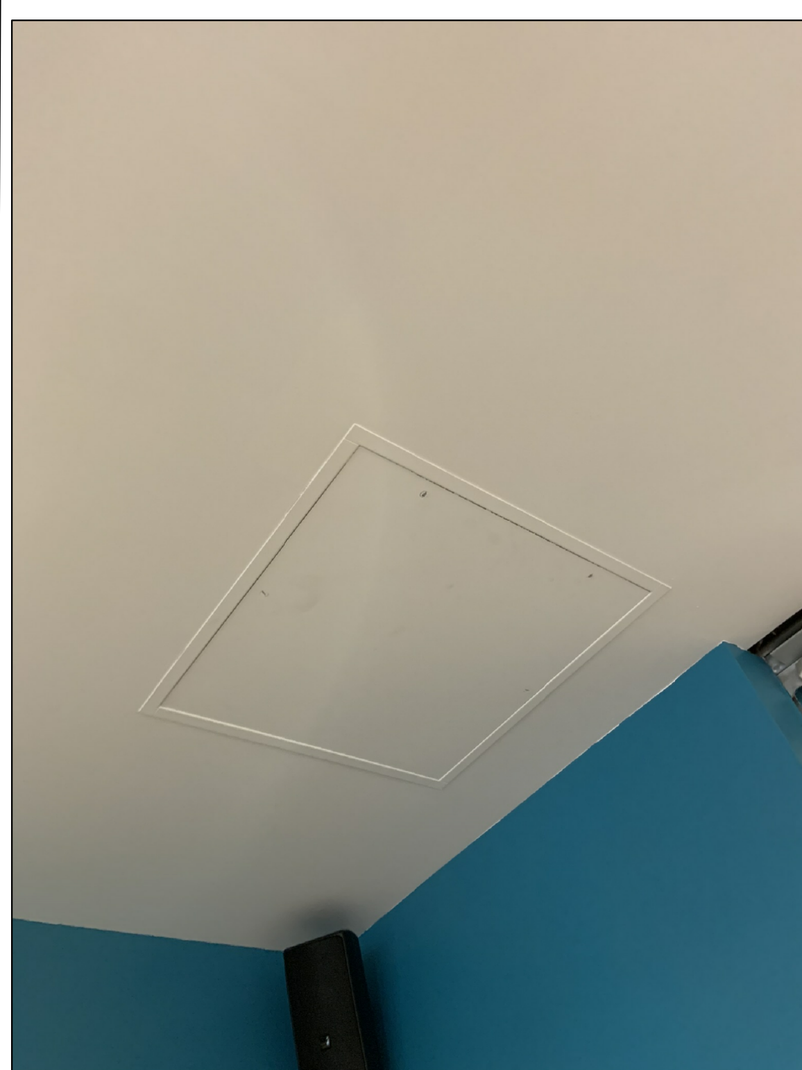
2 E1.1E EXISTING CEILING ACCESS PANEL NTS
