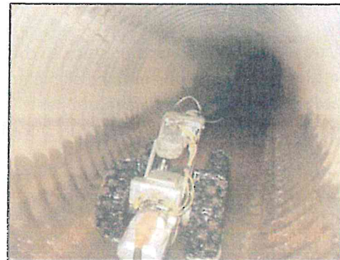
Typical CCTV Camera in Pipe
