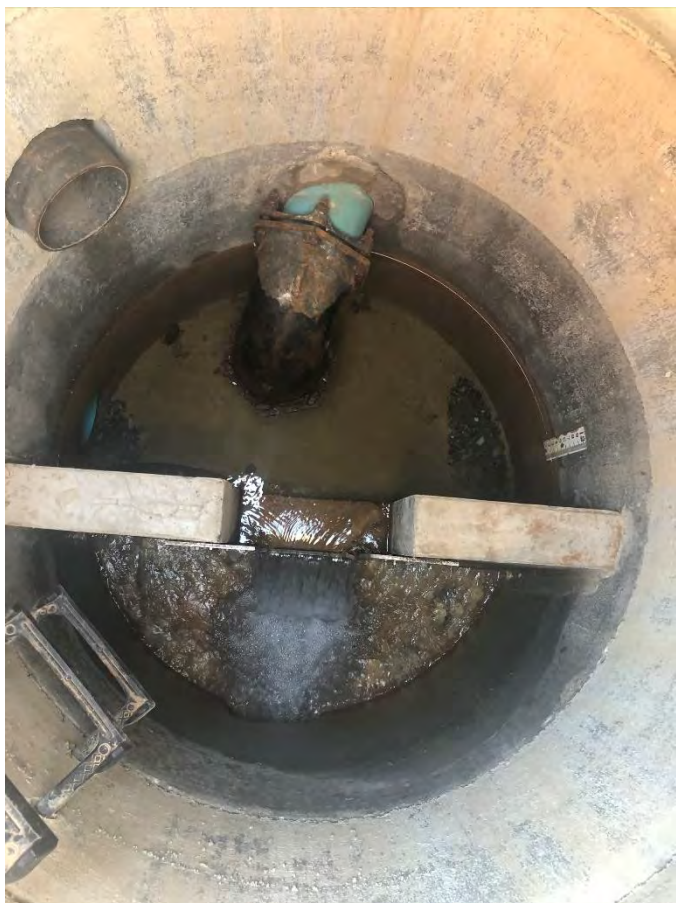
Photo 11- Spring 3 Collection box and weir
