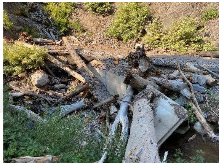
Damaged culvert terminus
