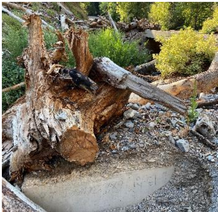
Exposed 6 x 4 culvert Dated 6-15-2001
