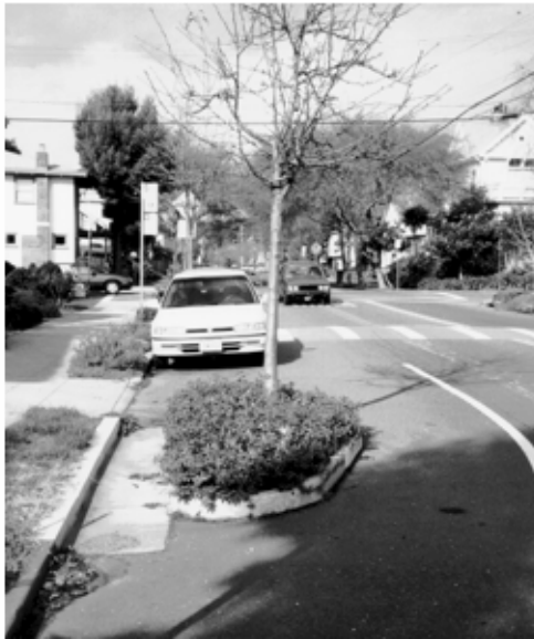
Figure 31. Pinch Points in Pavement
