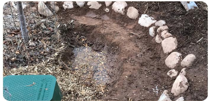
*Installing earthworks for a gravity-fed graywater system in Moab, UT (pipe outlet into green mulch shield). Credit - Roslynn Brain McCann*
