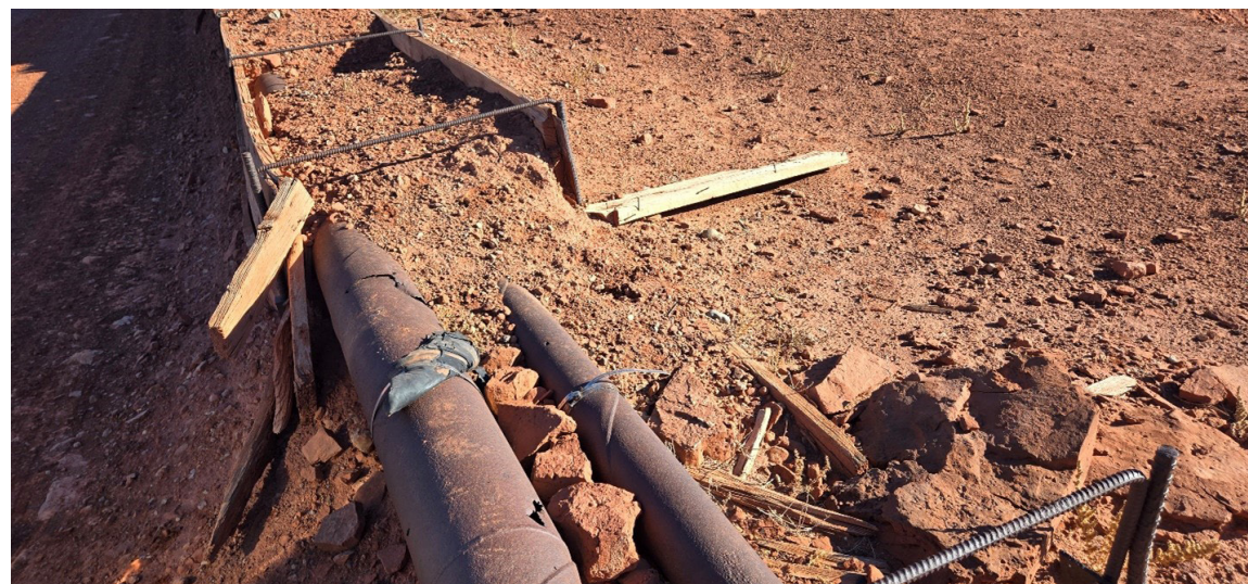
Figure 3 - Halchita Pipe Condition at Tanks
