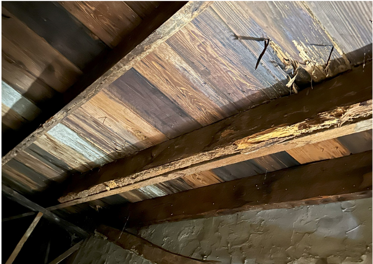
Photo 4 - View of damaged/deteriorated roof framing along south wall of rear room
