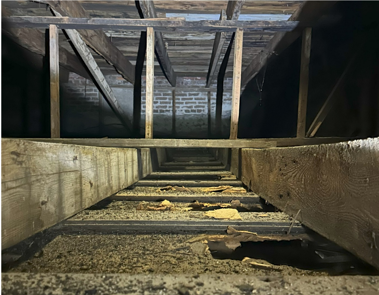
Photo 5 - View of damage/deterioration along ceiling framing from water intrusion at southwest corner of rear room
