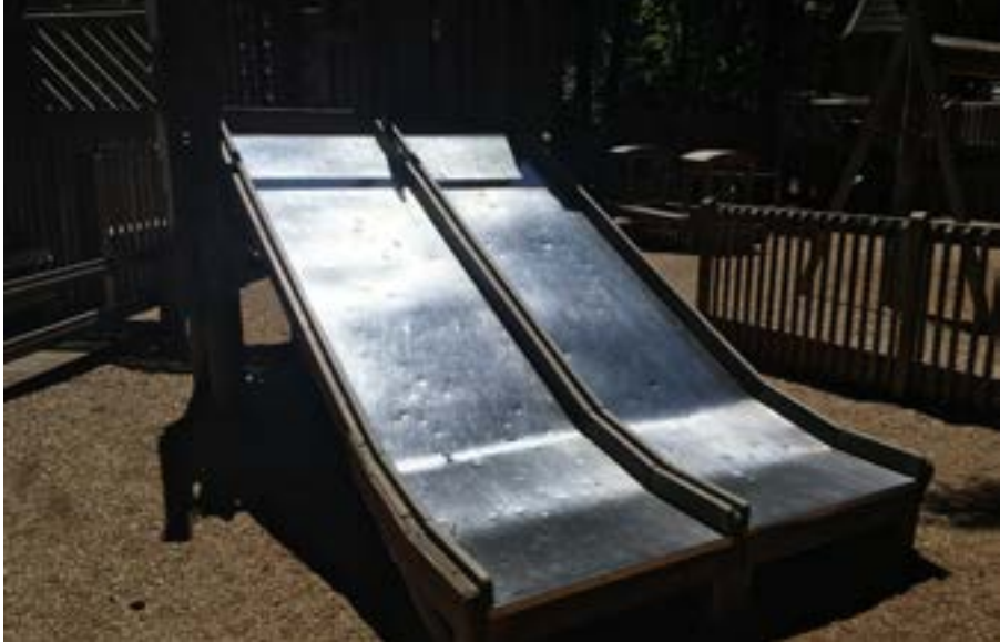
2. Deteriorating slide with loose composite sideboards
