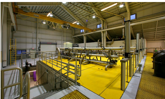
NLRSD WWTP Membrane Tanks
