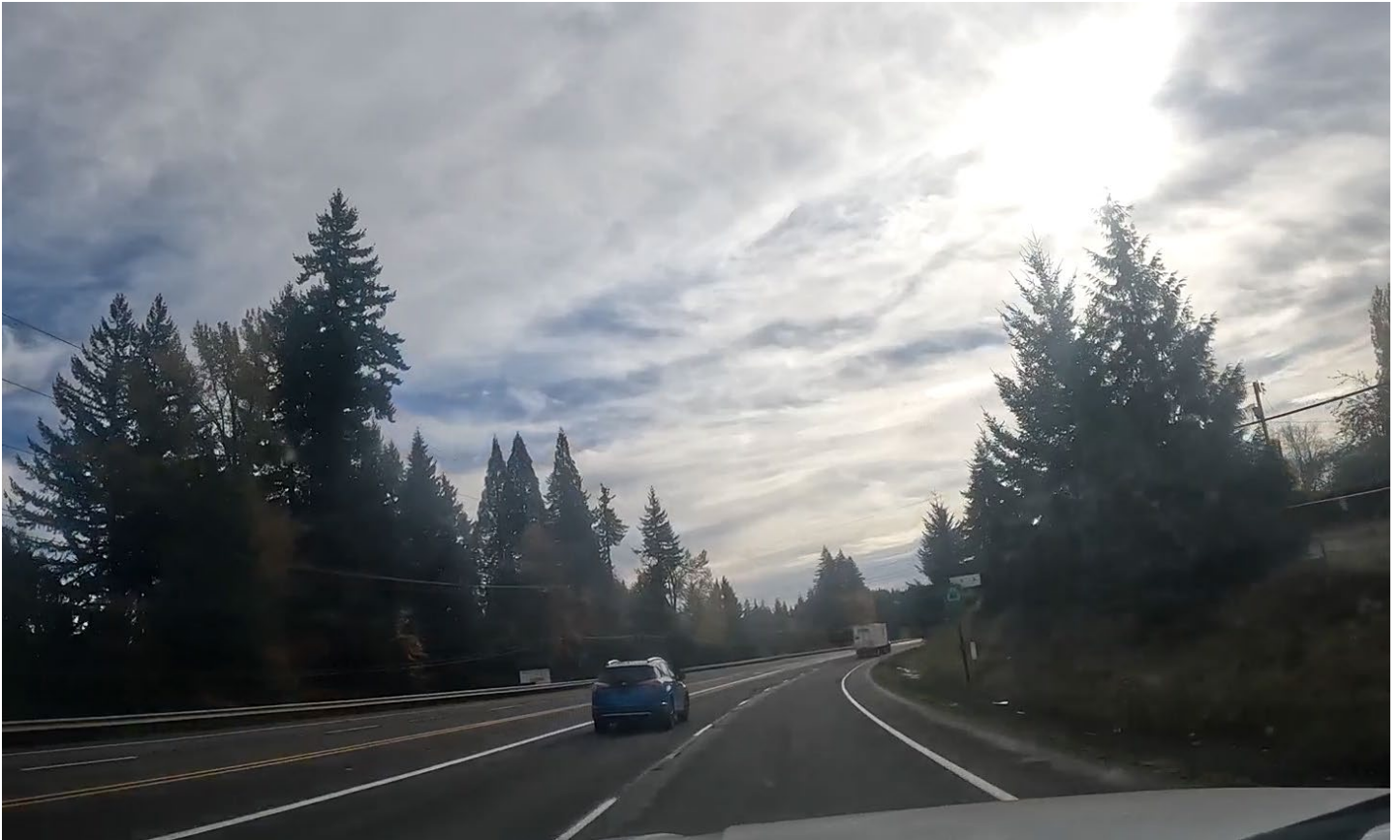
(15) Looking east from 350 feet west of SE Canyon Valley Road.
