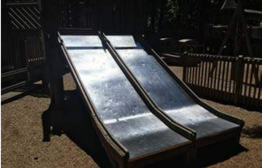
2. Deteriorating slide with loose composite sideboards
