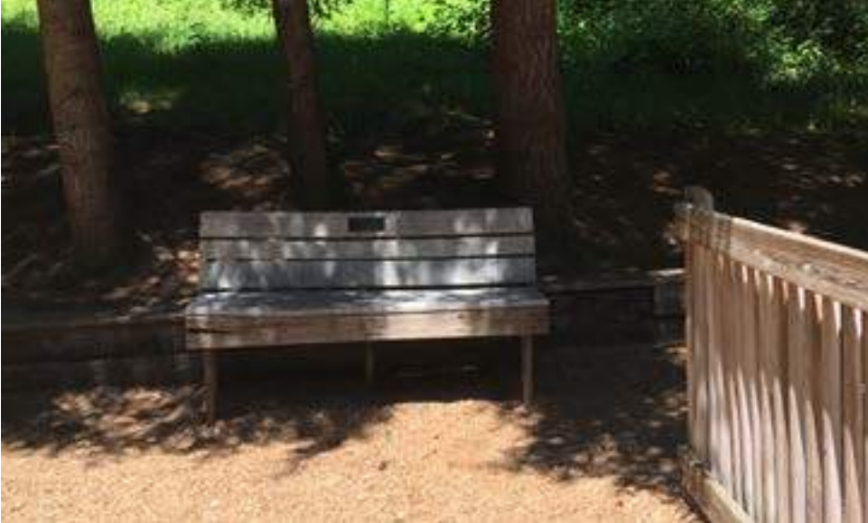
3. Park seating options are deteriorating, with wood rot and sinking planks
