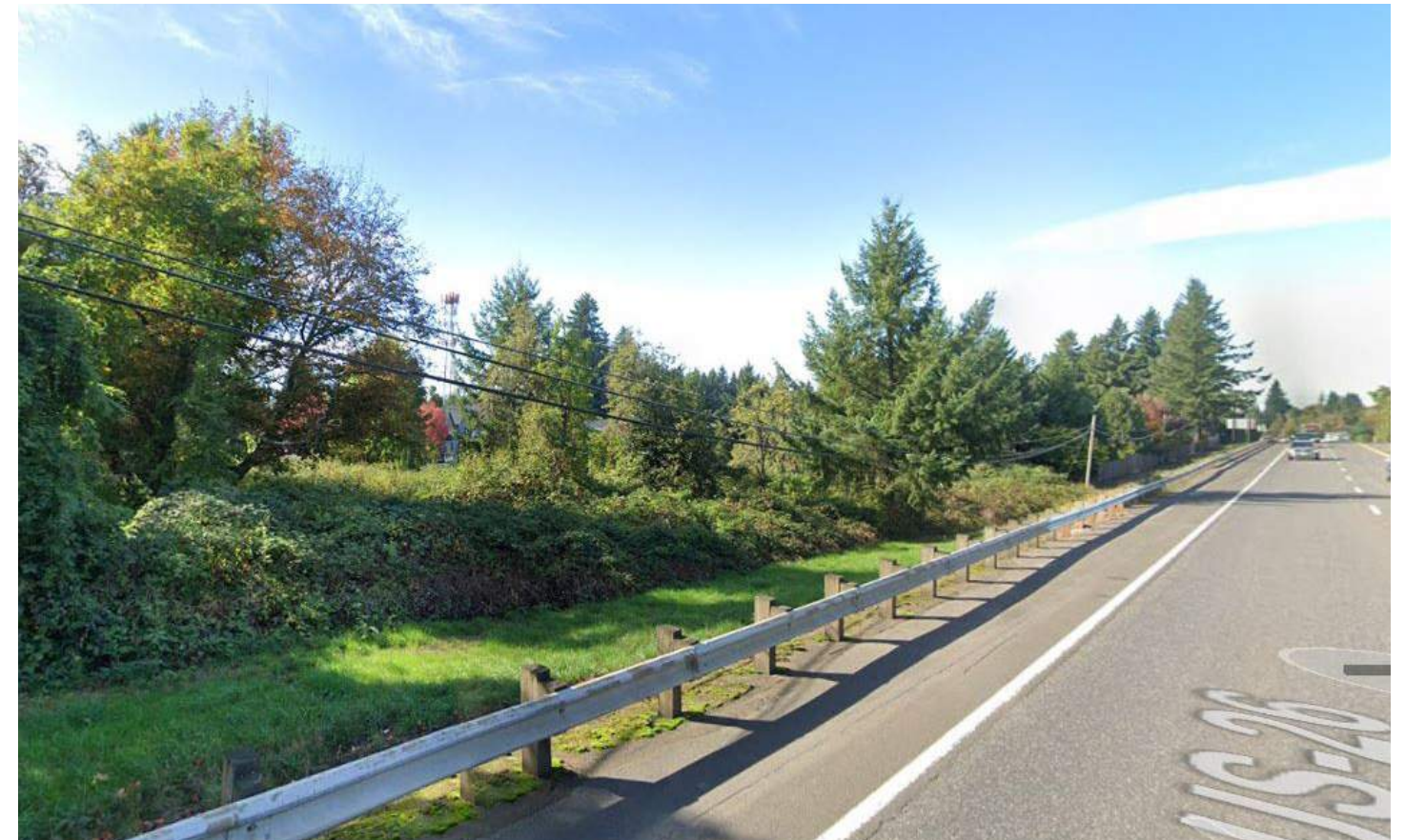
Highway 26 facing northwest
