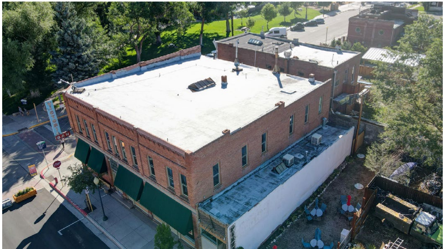
Roof View including one-story Cafe
