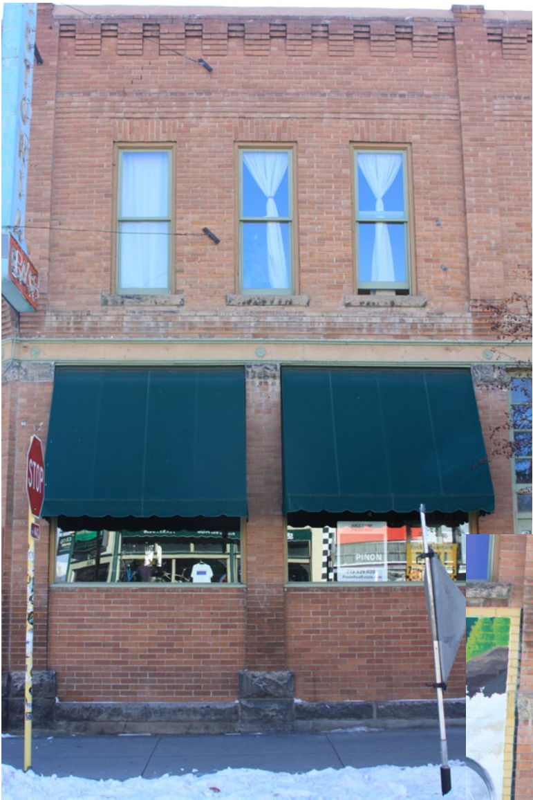
F Street brick infill windows
