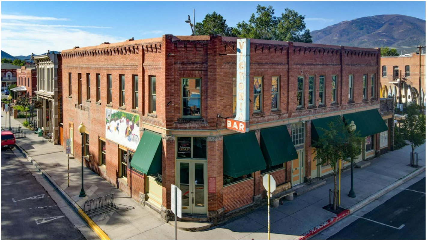
Corner View of the Victoria
