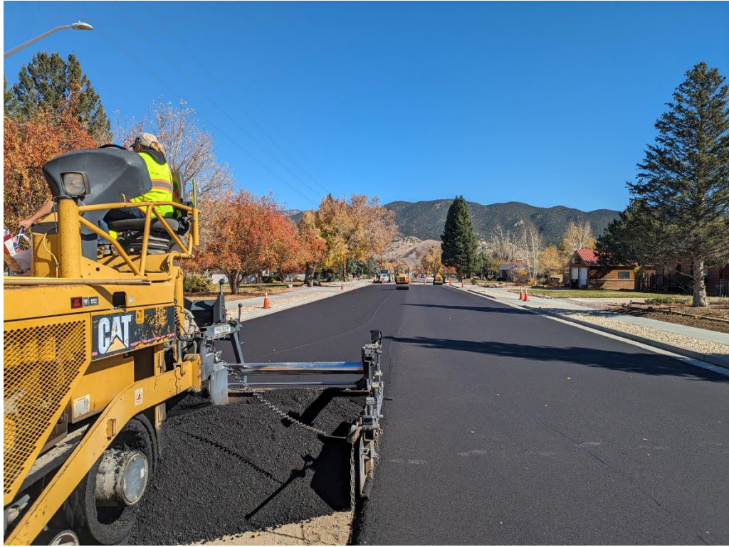
Figure 1 - Paving Phase 2 from Grant Ave. to Holman Ave.
