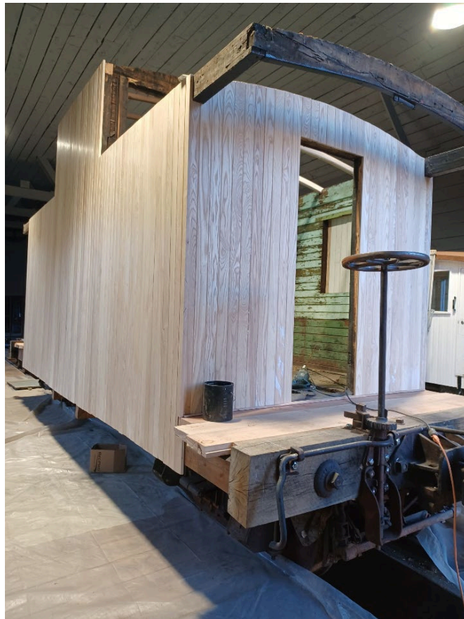
Figure 2 - Caboose Restoration in Silverton
