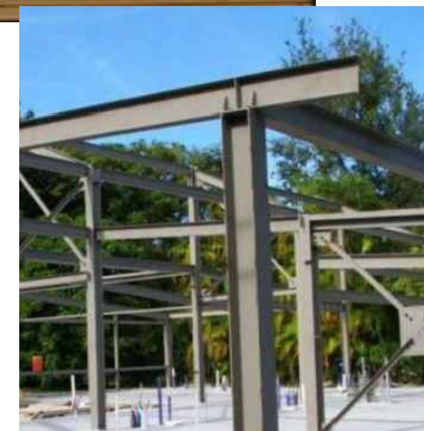
EXPOSED STRUCTURAL STEEL FRAME AT GROUND LEVEL
