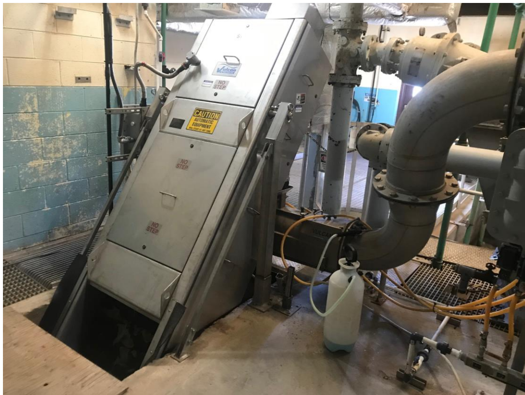
Figure 1 – Bar Screen Replacement
