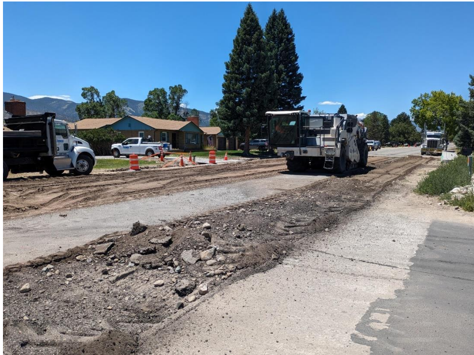
Figure 2 - Poncha Blvd. Asphalt Reclamation (FDR)
