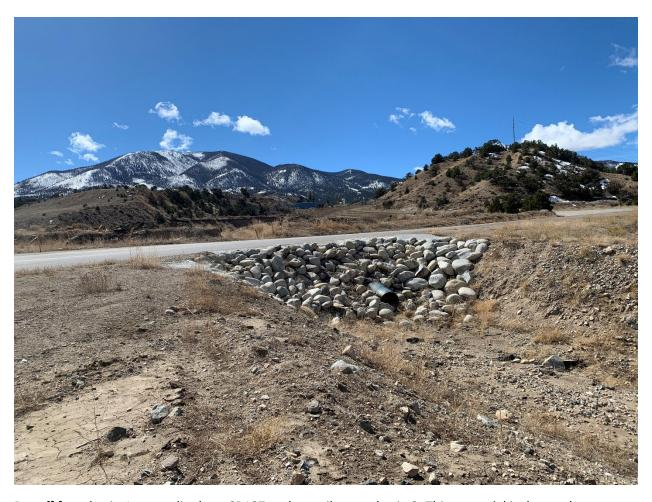
Runoff from basin 1 may split along CR107 and contribute to basin 2. This potential is due to the undersized culvert in the historic flow path at CR107, shown above. The undersized culvert should be addressed to prevent runoff from following CR107 from basin 1 into basin 2.
