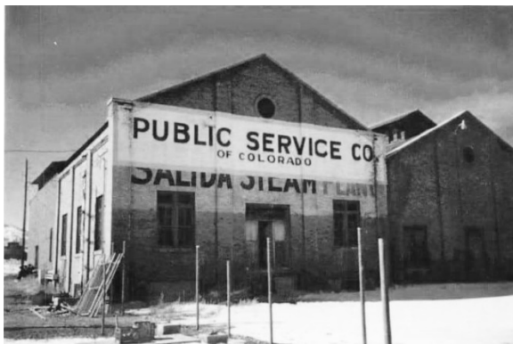
Photo 40: Edison Electric Light Plant, Salida Steam Plant (5CF.291)
