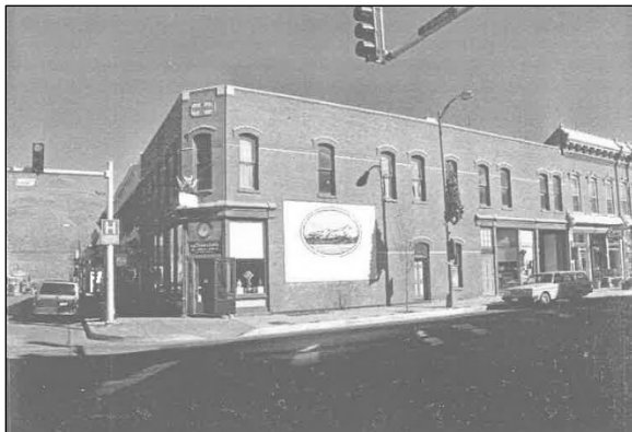
Photo 14: Twitchell Building, 101 N. F Street (5CF.406.45).
