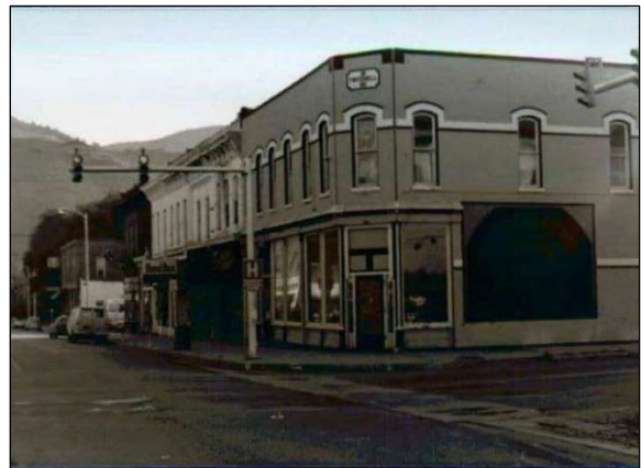
Photo 7: Twitchell Building, 101 N. F Street (5CF.406.45).
