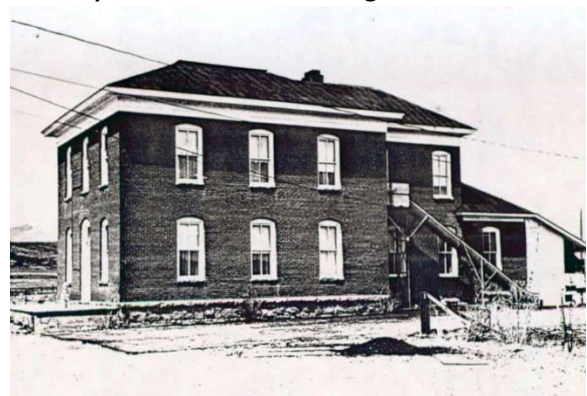
Photo 31: Chaffee County Poor Farm (5CF.190)
