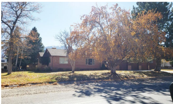
Photo 55: Post-WWII Ranch type residence, 525 Poncha Boulevard, built 1952.
