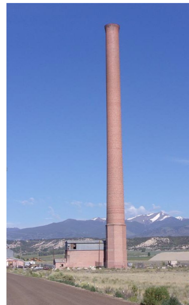
Photo 50: Ohio and Colorado Smelting Company Smokestack.
