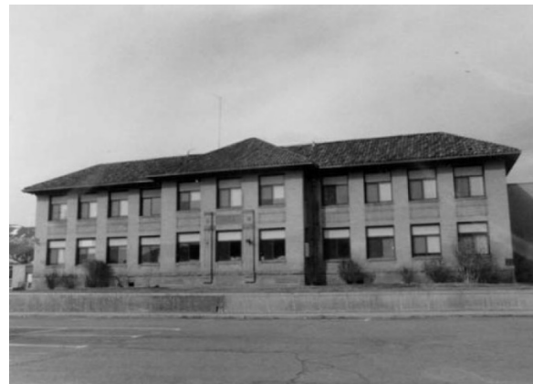
Photo 45: Kesner Memorial Building (5CF.1507)
