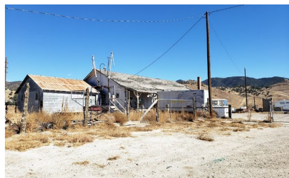
Photo 56: Chevron Oil Storage Building, built 1951. Located at the railroad crossing of County Road 175.
