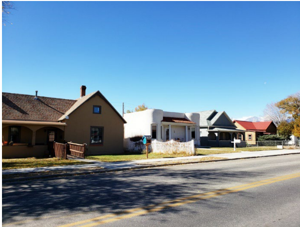
Photo 78: 605 West 1 st Street
