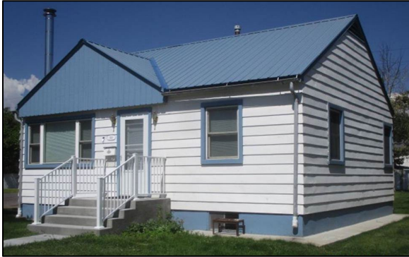
Photo 63: Minimal Traditional type house at 948 G Street (Source: Chaffee County Assessor)
