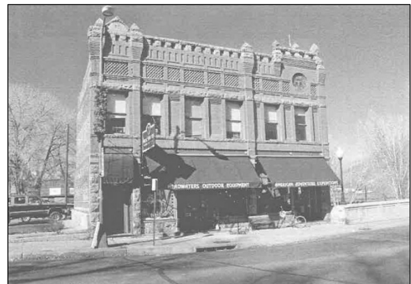
Photo 16: Bon Ton/Manhattan Hotel, 228 N. F Street (5CF.213).
