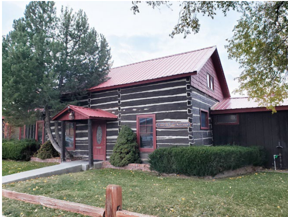
Photo 46: Example of pre-1880's square-hewn log construction, 1604 H Street.
