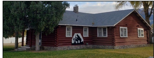
Photo 66: Rustic style American Legion Building at 235 West 10 th Street
