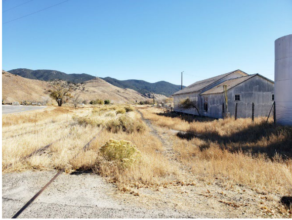
Photo 47: D&RG tracks originally constructed in 1880 between Texas Creek and Leadville with Salida as the major junction. Photo taken at County Road 175 crossing north of town.
