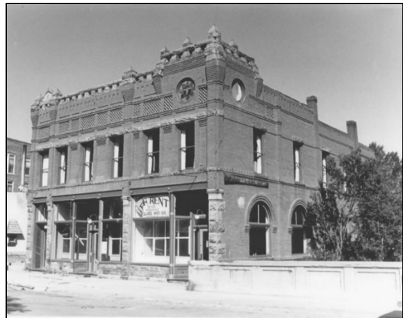
Photo 58: Manhattan Hotel (Source: NR Nomination)
