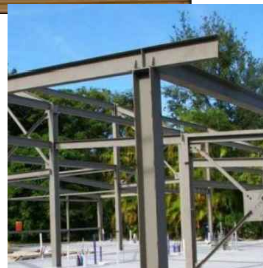
EXPOSED STRUCTURAL STEEL FRAME AT GROUND LEVEL
