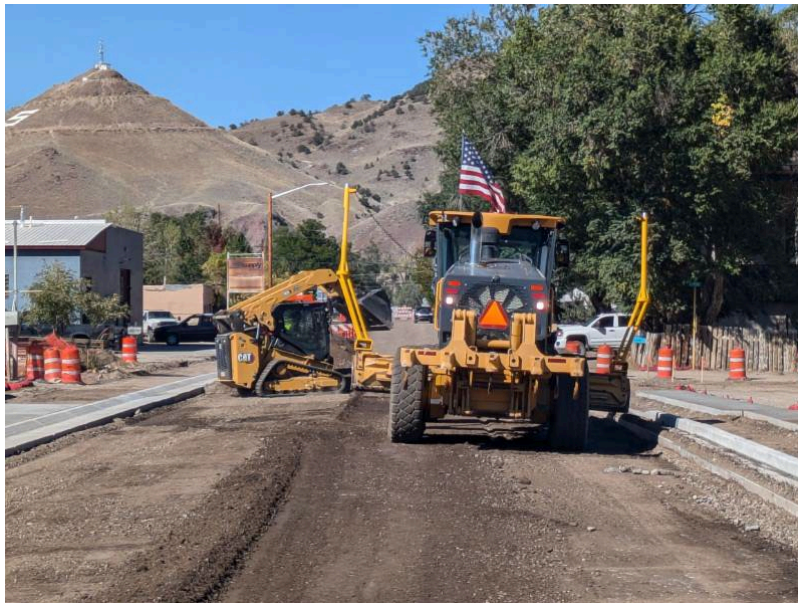
Figure 3 - Oak Street Prep for Paving
