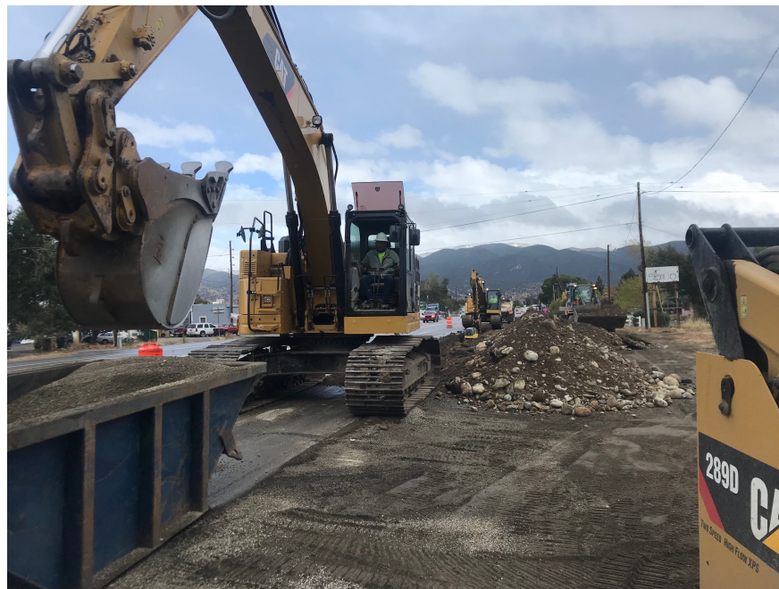
Figure 1 – Low Zone Waterline Replacement
