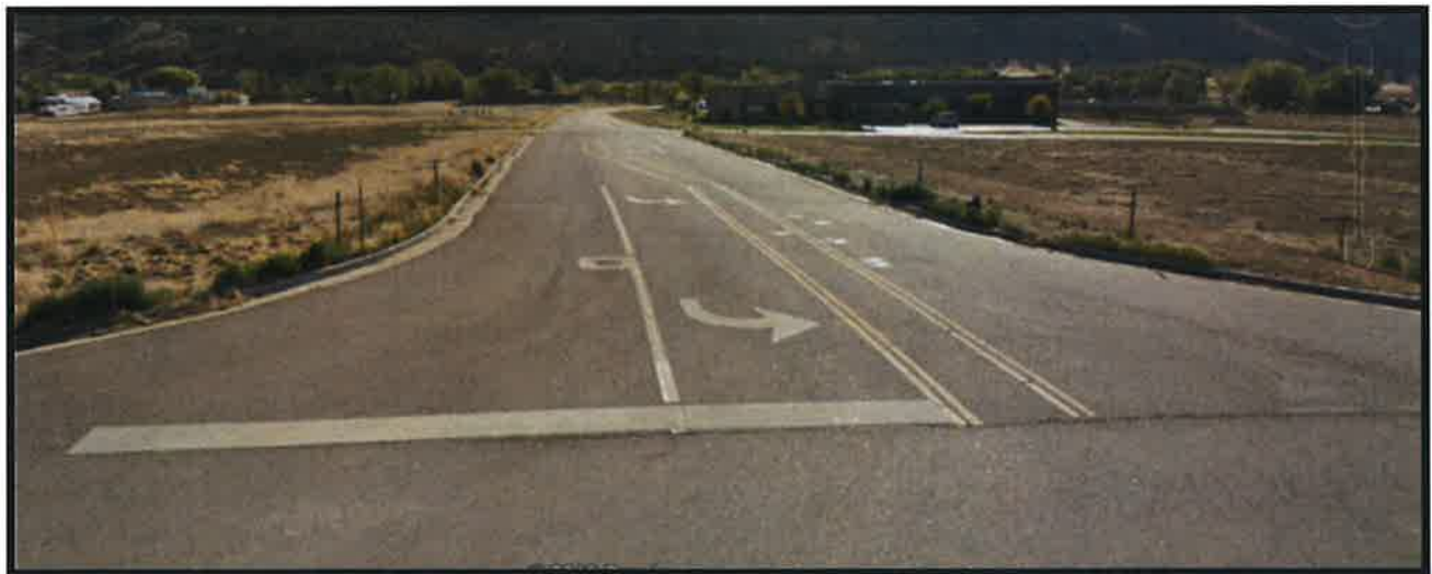
Figure 9-Vandaveer Ranch Road looking East from Highway 50
