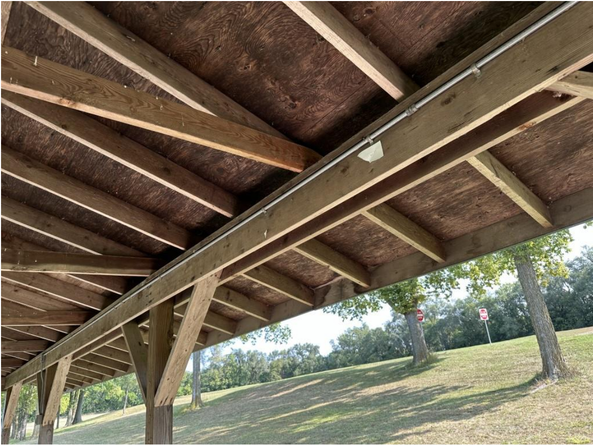
Photo 07 - Typical Beams To Posts
