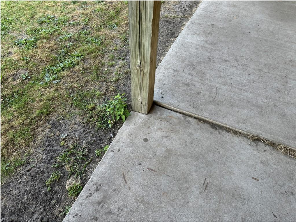
Photo 09 - Slab Step At Post
