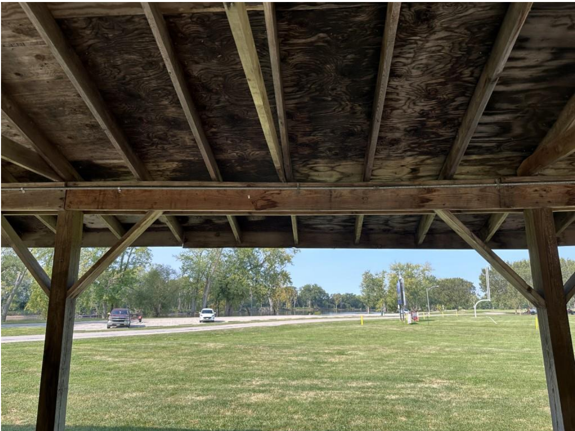
Photo 08 - Roof Beams At Settled Posts
