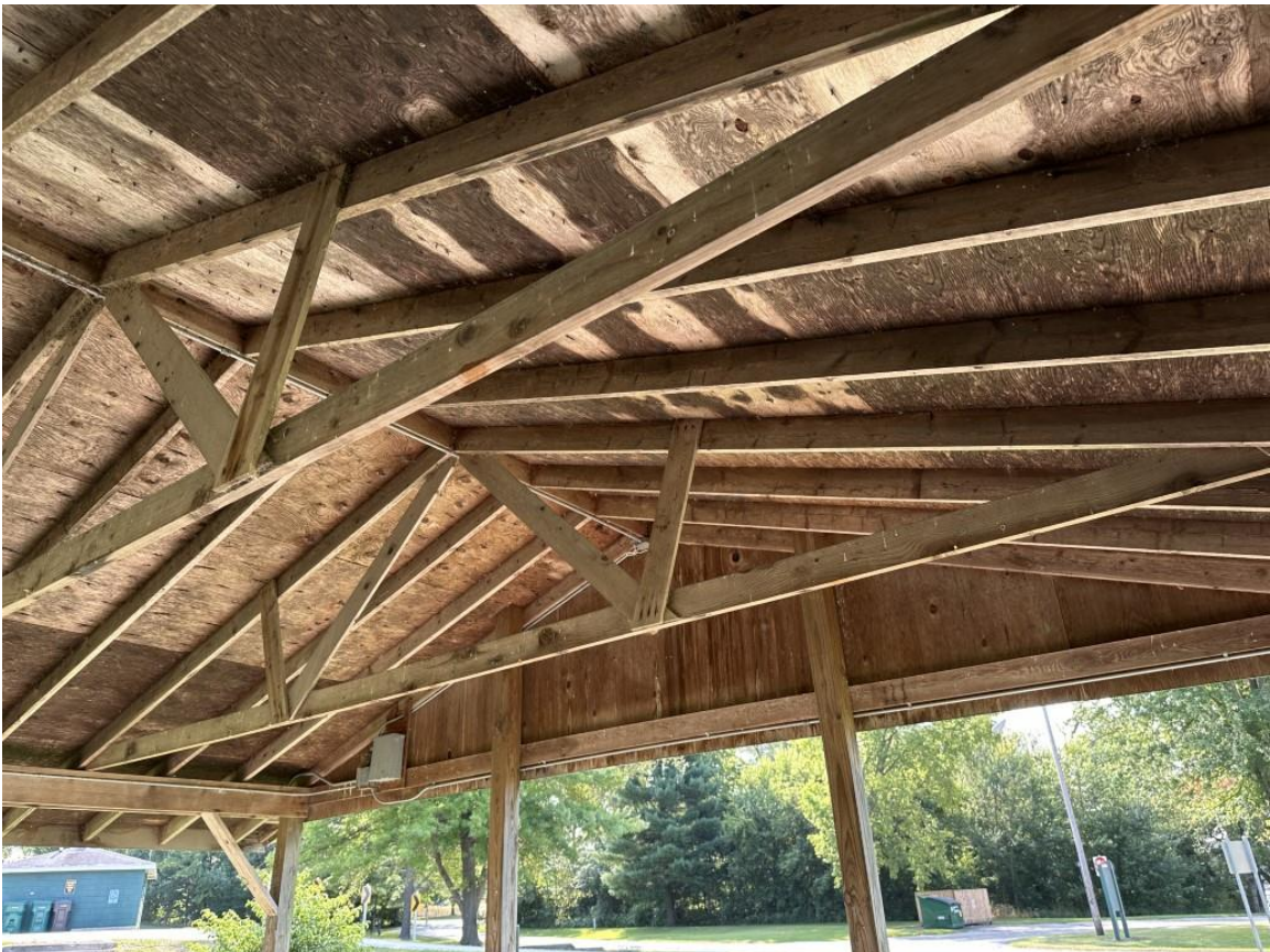
Photo 06 - Interior Trusses
