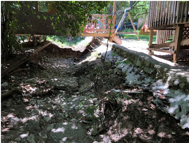
Figure 1 – Channel between 303 and 2910 Hatley Drive (facing upstream)
