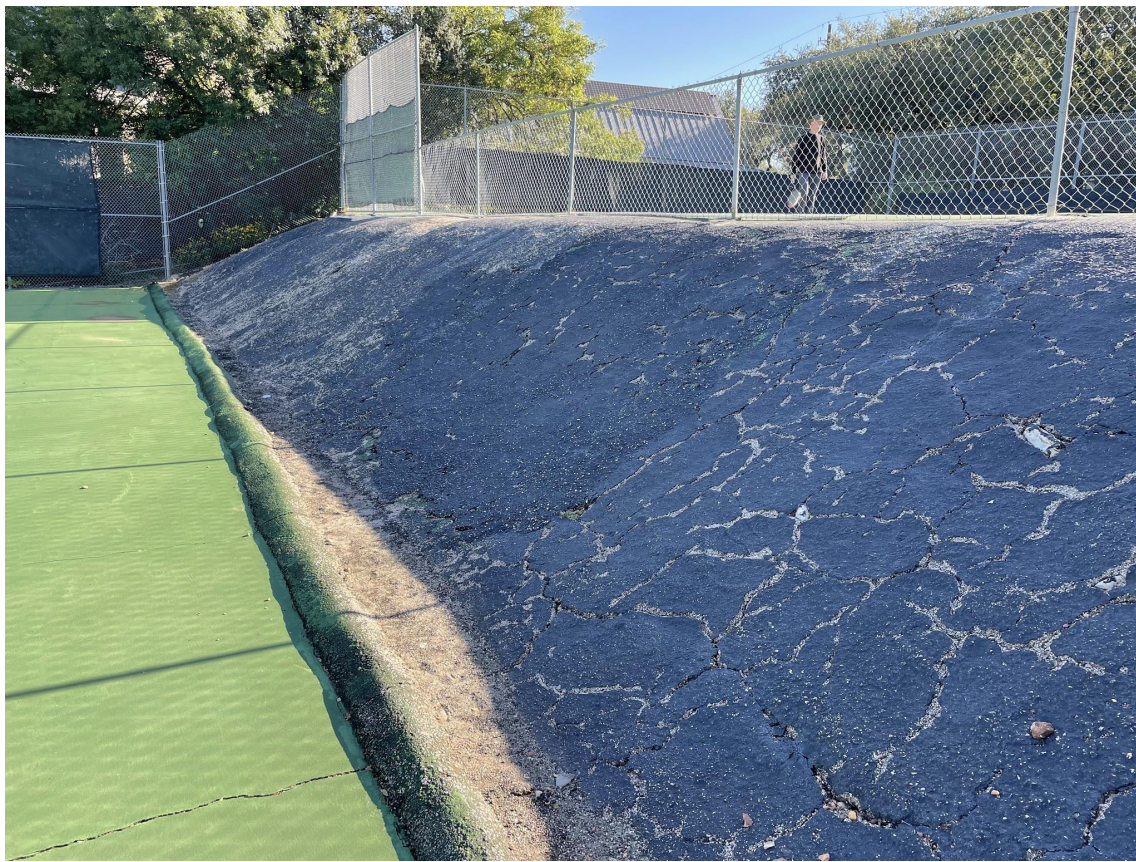
Asphalt berm between lower and upper courts: wider than needed barrier; unsightly
