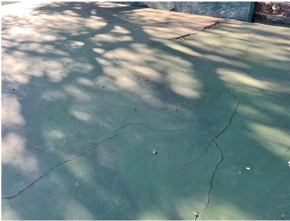
Lower court damage : multiple cracks (some dangerous), worn surface
