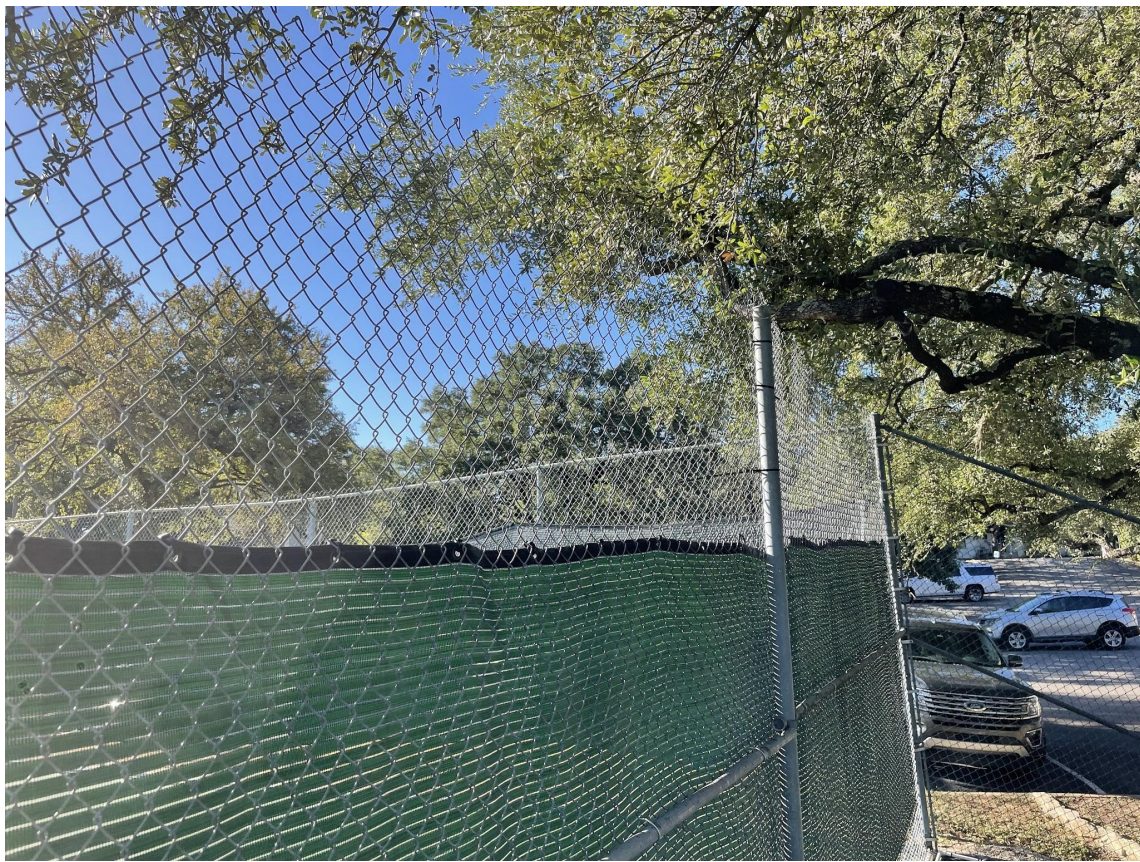
Chain link fence : rusted, leaning, and missing rails and other parts
