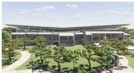
Dripping Springs Community Library
