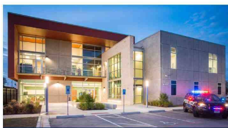
Georgetown Public Safety Center
