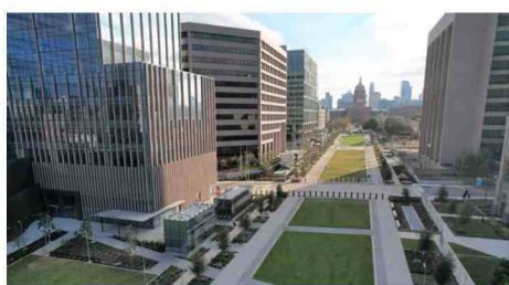
TFC Capitol Complex, Phase 1
