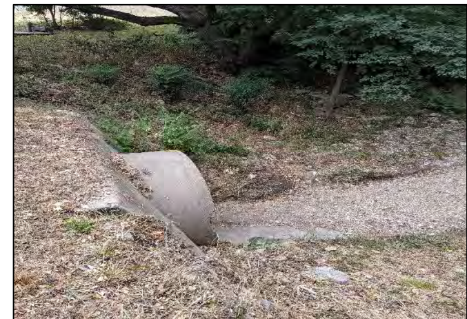
Pleasant Cove culvert crossing, upstream. 09/11/2019
