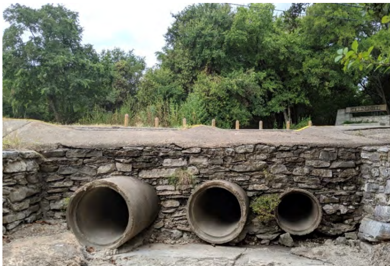
Figure 1: Edgegrove Drive Low Water Crossing (September 11, 2019)
