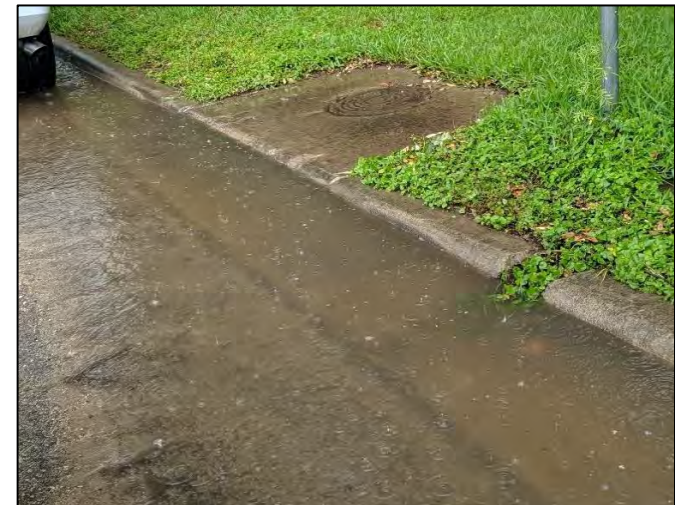
Pond inlet during rain event. 06/06/2019
