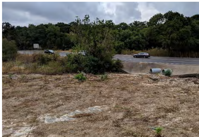
Figure 5: Bee Caves Road Culvert, Downstream (September 11, 2019)
