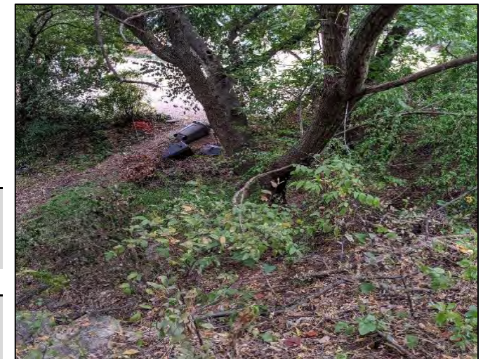
Ravine at 4803 Timberline Drive. 09/11/2019
