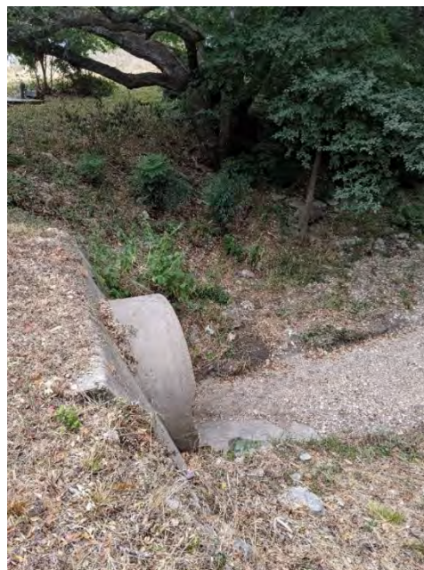
Figure 7: Pleasant Cove Culvert, Looking Northeast/Downstream (September 11, 2019)
