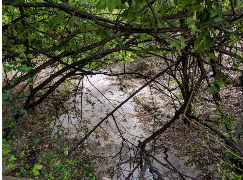
Figure 6: Rockway Cove Culvert, Looking Southwest/Upstream (September 11, 2019)
