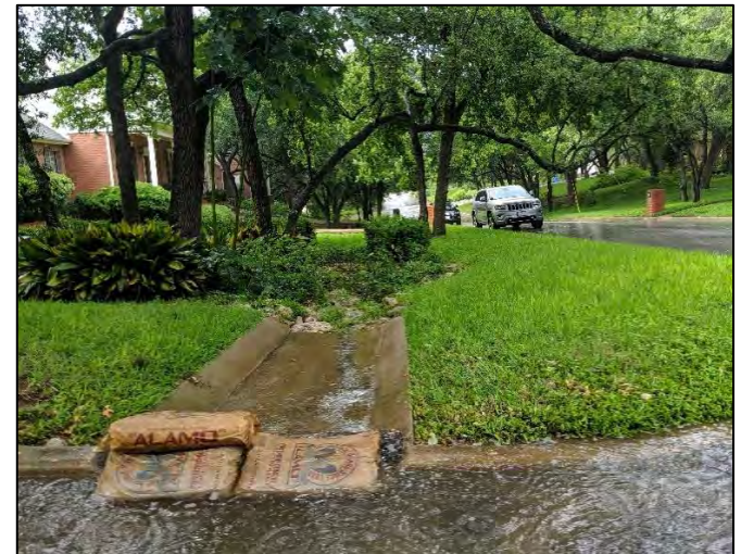
200 Wallis Drive, during rain event. 06/06/2019
