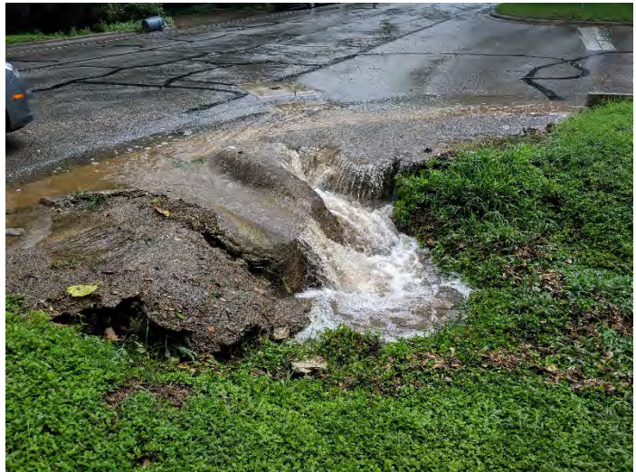
Figure 4: Nixon Drive Culvert, Looking Southeast/Downstream (June 6, 2019)
