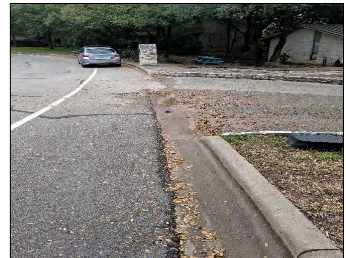
Timberline Drive looking northeast. 09/11/2019
