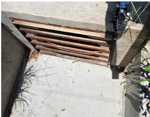
Figure 6 – Recently installed safety screen on the upstream headwall conveying flow across Bettis Blvd toward 307 Inwood
