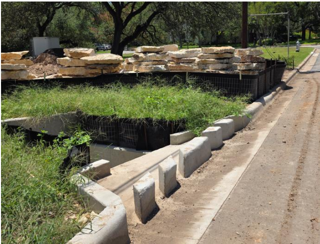
Figure 4 – Recently installed curb cut on Bettis Blvd., facing upstream to the northwest.
