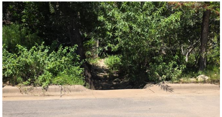
Figure 7 - Bettis Blvd curb cut downstream side (facing east)
