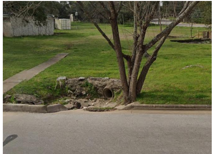
Figure 5 - Bettis Blvd curb cut prior to the recently installed drainage infrastructure (February 2024).
