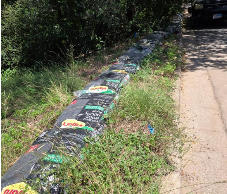
Figure 8 - Bags of Mulch placed to increase berm height and mitigate curb overtopping
