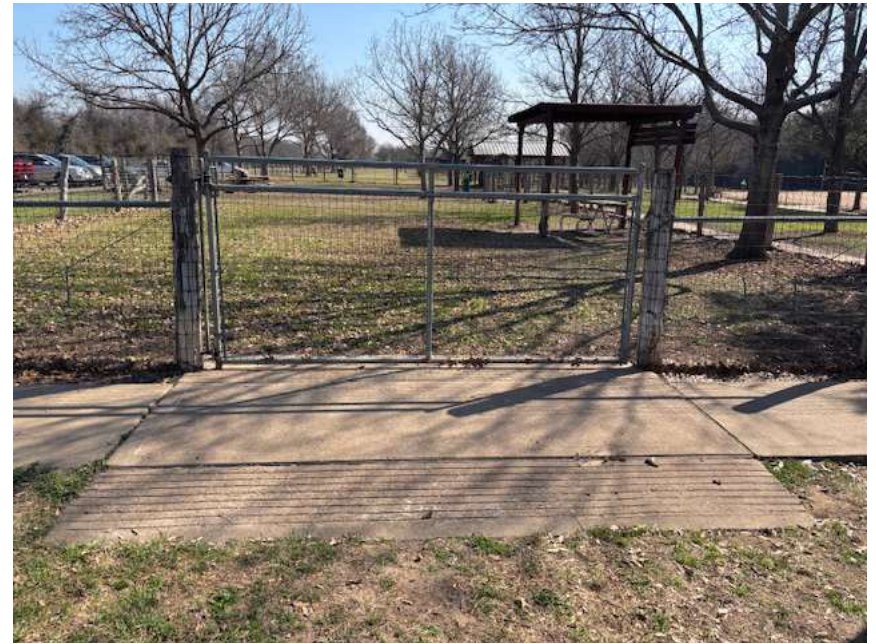
Maintenance entrance with shade structure in background
