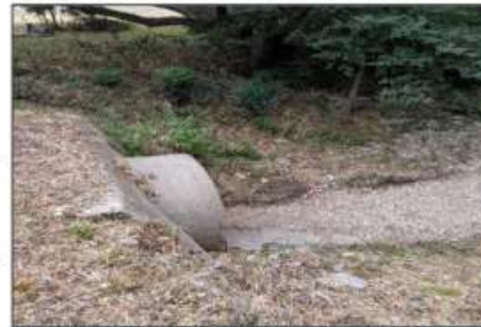
Pleasant Cove culvert crossing, upstream. 09/11/2019
