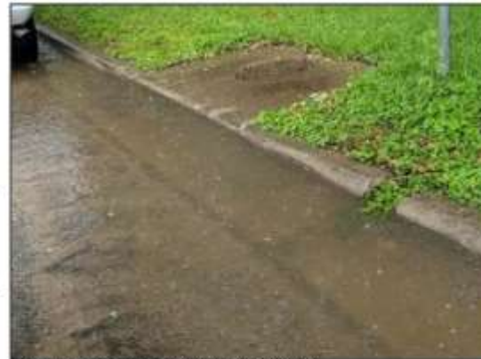
Pond inlet during rain event. 06/06/2019
