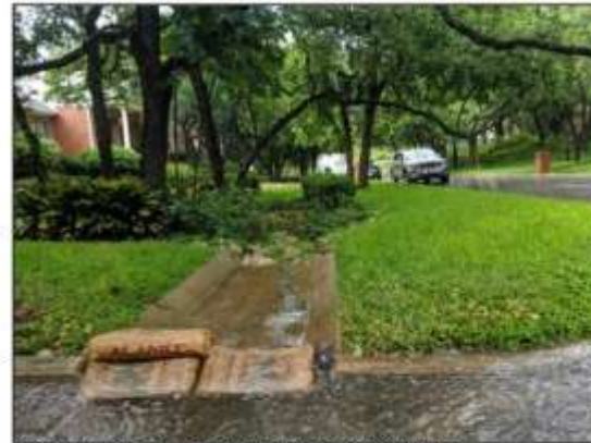
200 Wallis Drive, during rain event. 06/06/2019
