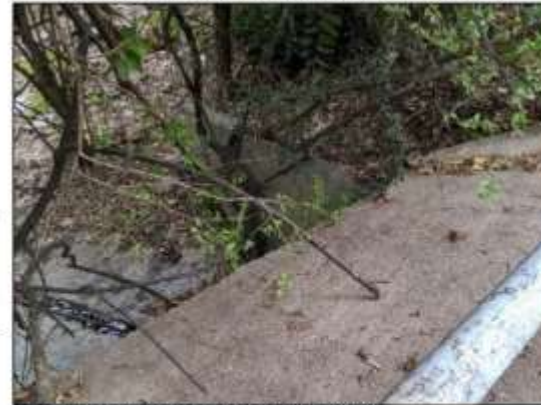
Outfall at Town Lake tributary. 09/11/2019
