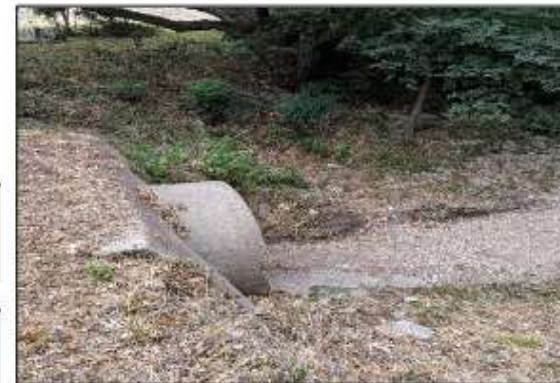
Pleasant Cove culvert crossing, upstream. 09/11/2019
