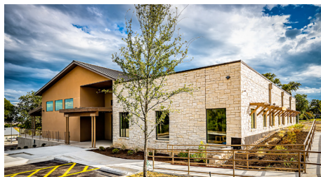
CASA Training and Support Center
