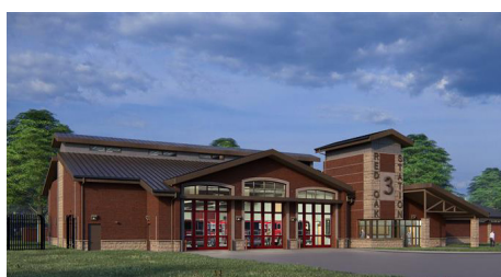
Red Oak Fire Station No. 3
