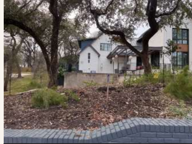
From curb looking up — steep grade change; pool exposed above existing wall
