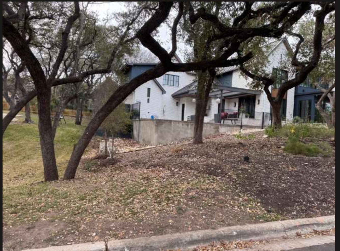
View from street — curved lot, slope & exposed pool wall visible · Laura Lane, Rollingwood TX
