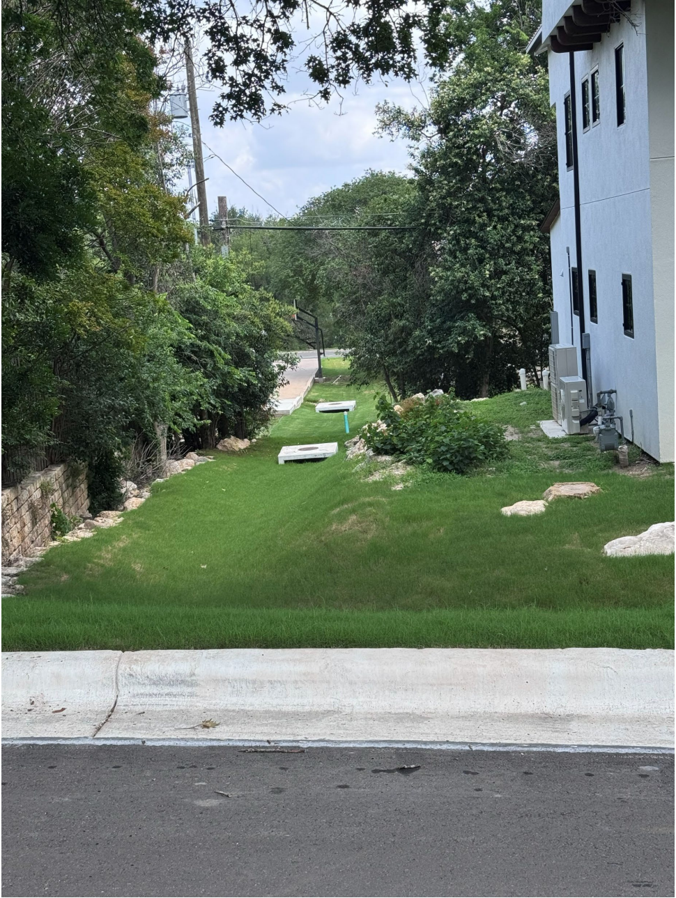
EASEMENT NORTHWEST SIDE 1
