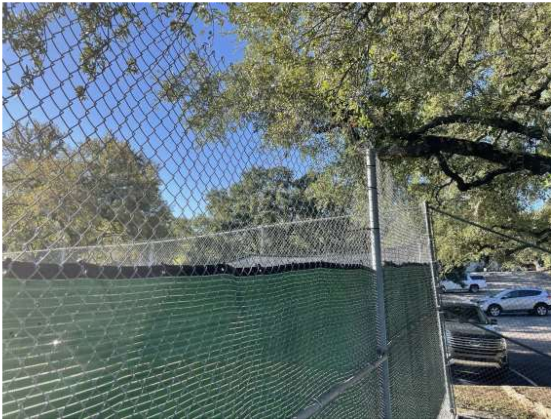
Chain link fence: rusted, leaning, and missing rails and other parts
