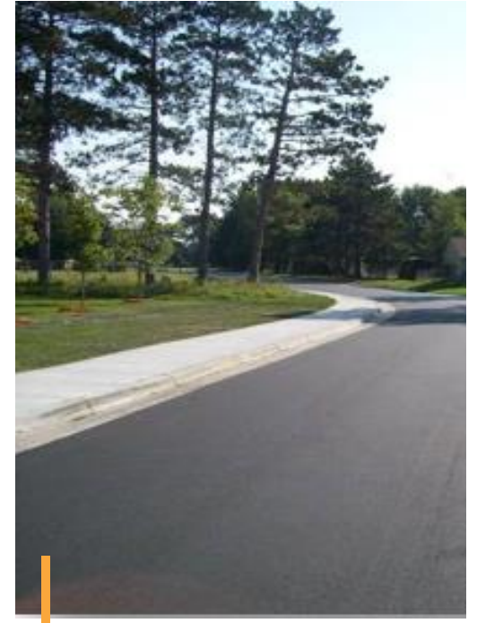
Reconstruction Typical for Failing Roadways
