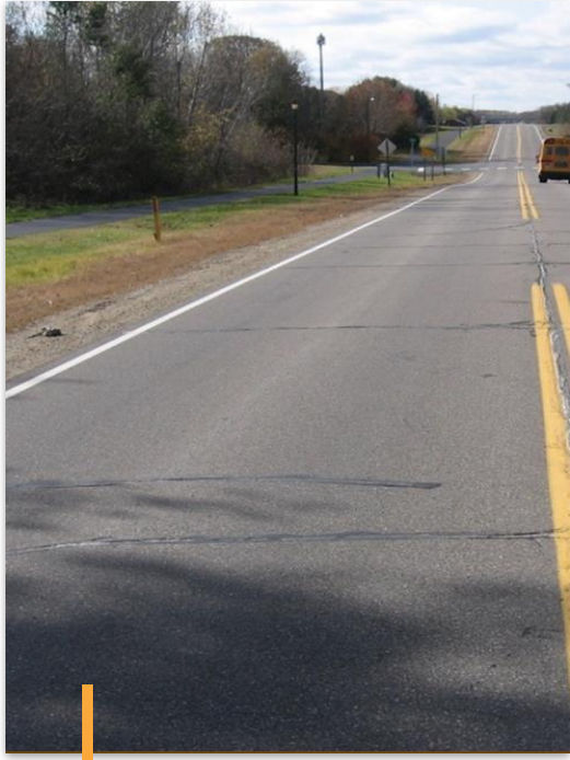
Corrective Maintenance Typical for Excellent & Good Rated Roadways
