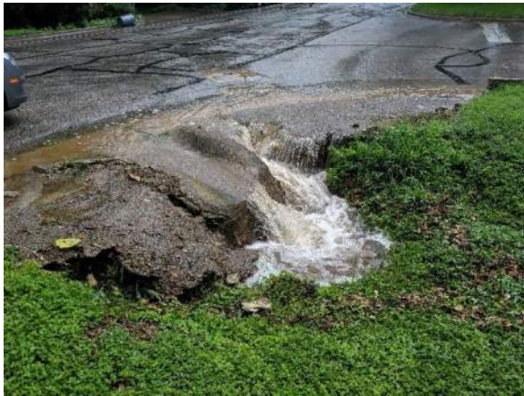
Figure 3 – Culvert at 300 Pleasant Drive Northwest towards Nixon/Pleasant Intersection
