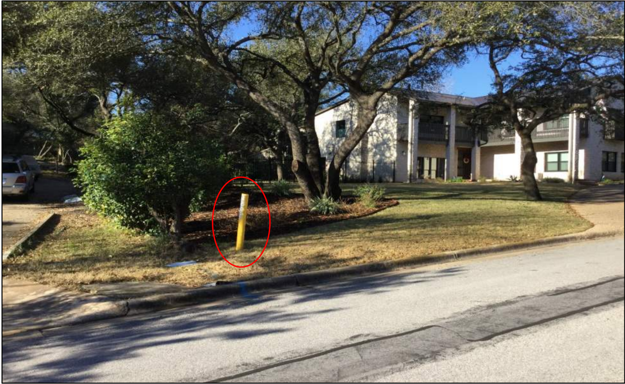
Photo 9: Viewing natural gas pipeline indicator on Pleasant Drive at northeastern portion of the Review Area.
