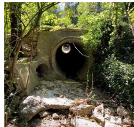
Figure 14 – 18-inch and 54-inch Culverts at Pleasant Cove Facing West
