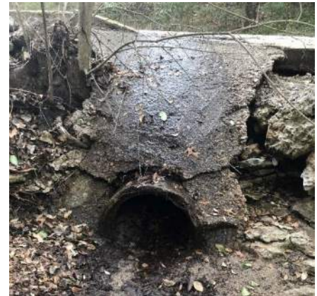
Figure 13 – 18-inch Culvert on Nixon Drive Facing Northwest
