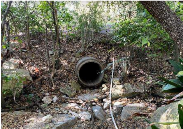
Figure 9 – Downstream of 20-inch RCP, between 303 and 305 Nixon Drive Facing Northwest
