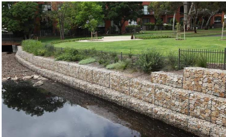
Figure 16: Rock Gabion Wall Lined Channel with Guardrail
