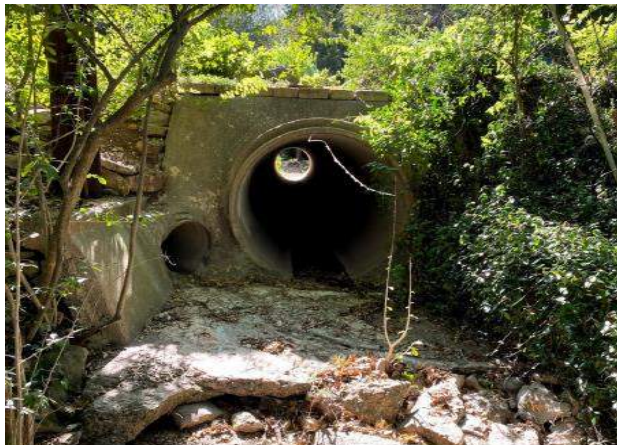
Figure 7 – Downstream of Pleasant Cove 18-inch and 54-inch RCP, Facing West
