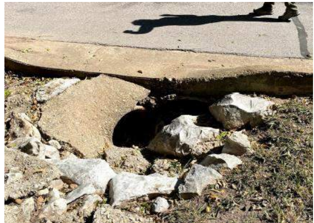
Figure 12 – Upstream 310 Pleasant Drive Culvert Facing Southeast
