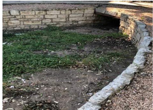
Figure 8 – Downstream of 301 Pleasant Drive Private Culvert, Facing Northwest
