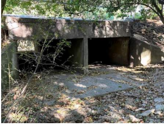
Figure 1 – Upstream side Hatley Drive Culvert Facing Northeast
