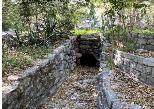
Figure 10 – Upstream of 305 Pleasant Drive Facing Northwest
