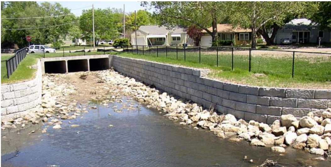
Figure 15: Dry Stacked Limestone Wall Lined Channel with Guardrail
