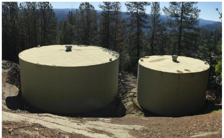
Figure 1. A pair of welded steel tanks make up the clearwell for the Colfax water system. Both tanks have PAX Water Mixers and PAX Powervents (visible on the top of each tank).
