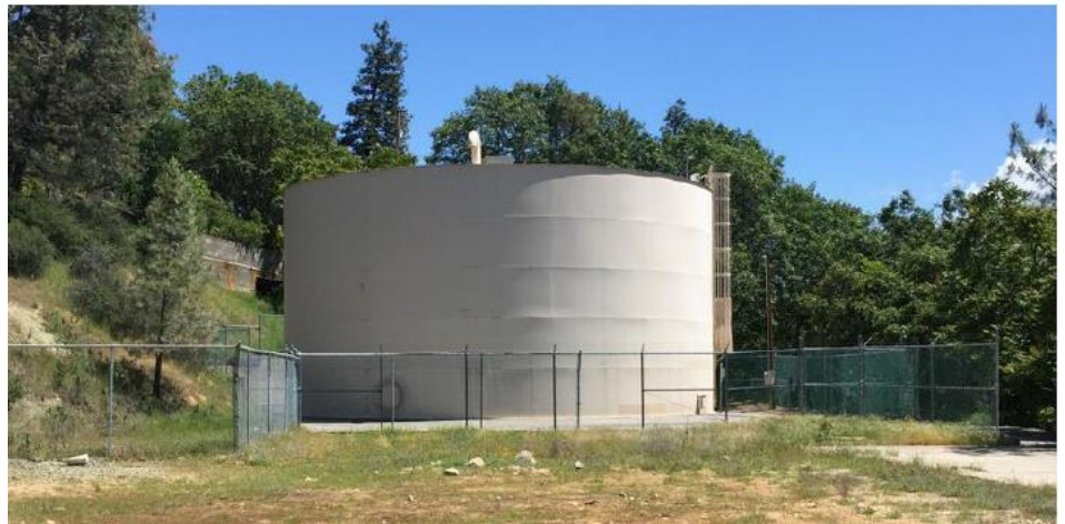
Figure 2. The 600,000-gal Ballpark Tank had a PAX Water Mixer and PAX Powervent.
