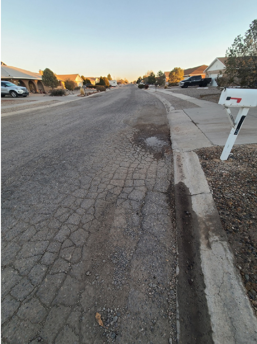
Figure 3: Alligator cracking
