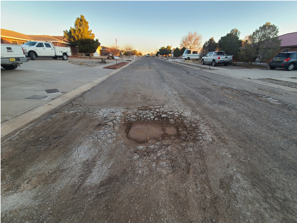
Figure 1: Subgrade exposure
