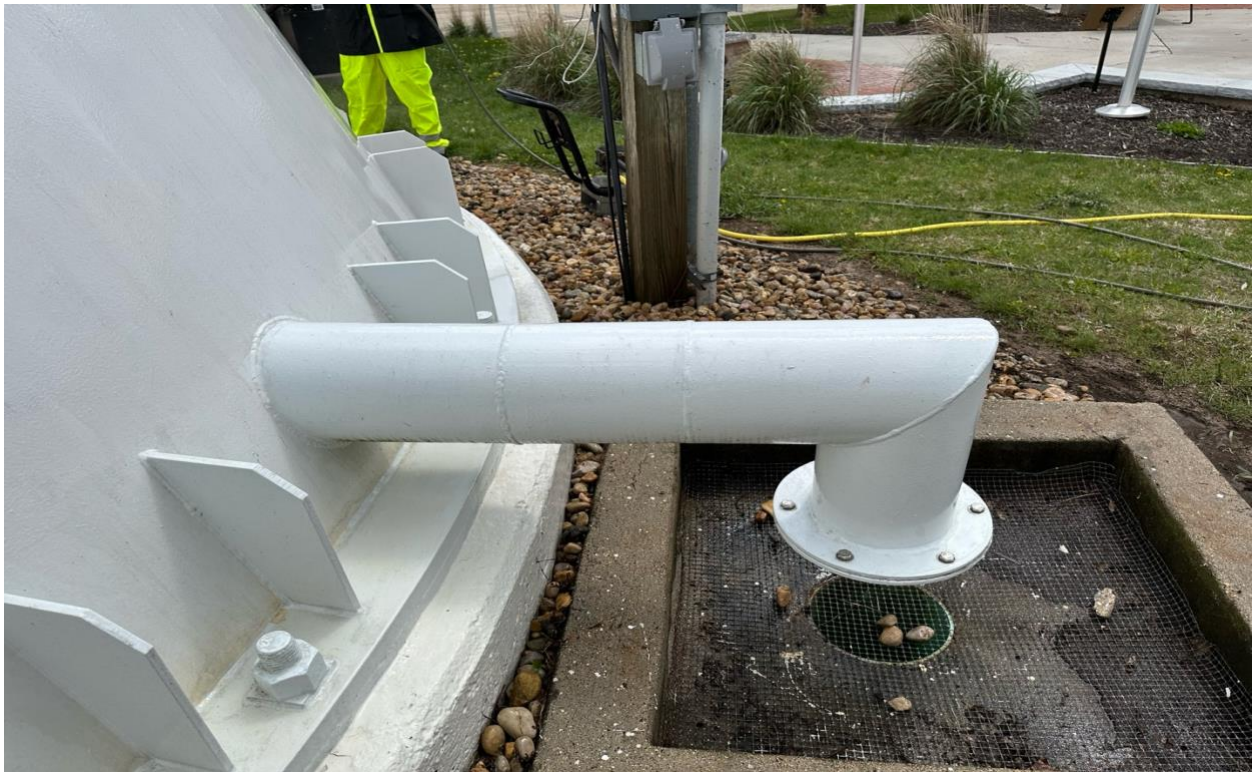
Base Cone After Power Washing
