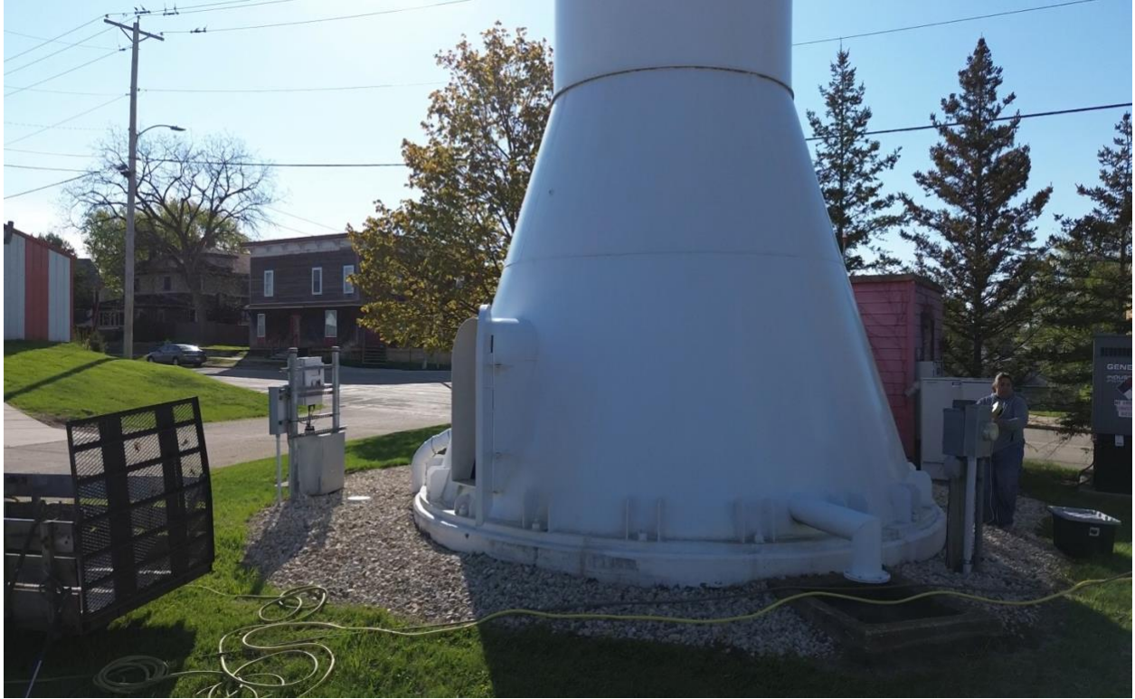
Base Cone Before Power Washing
