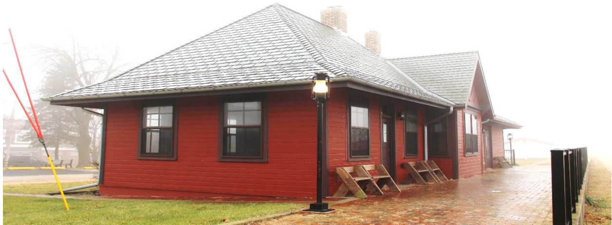
AHI No. 64662, Chicago and Northwestern Depot, side (east) elevation and front (north) facade, facing southwest. Project improvements include repaving the existing path located along the side of the depot.
