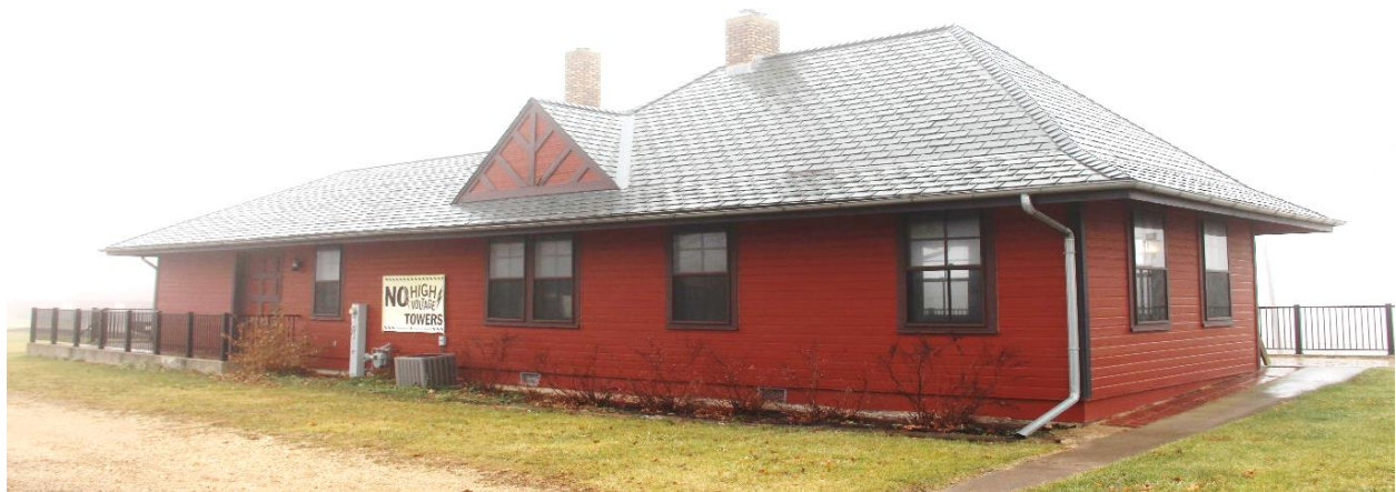
AHI No. 64662, Chicago and Northwestern Depot, rear (south) and side (east) elevations, facing northwest. Project improvements include repaving the existing path located along the side of the depot.
