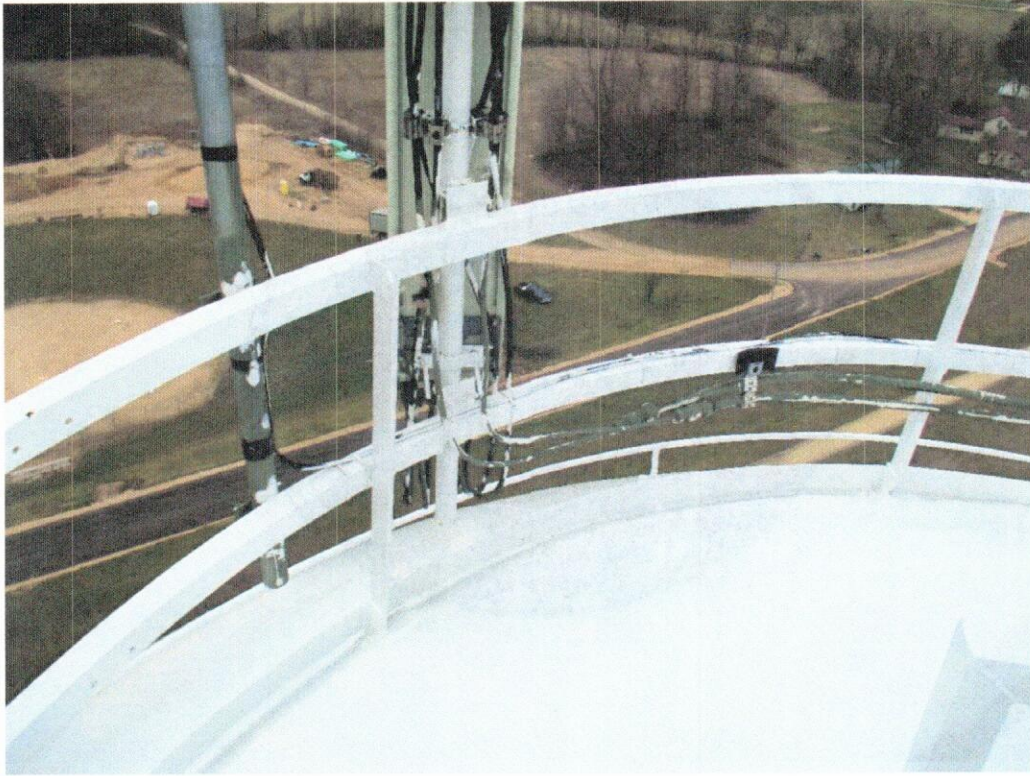
Exterior Roof and Handrail – Good Condition
