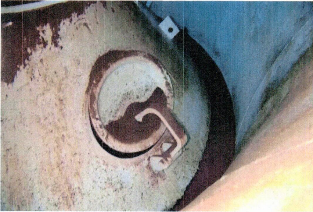
Interior Wet Access Hatch - Good Condition - Minor Sediment
