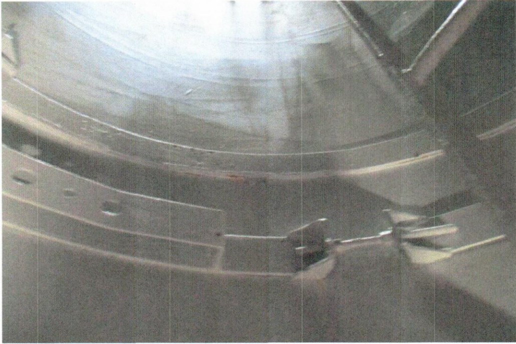
Access Tube – Good Condition
