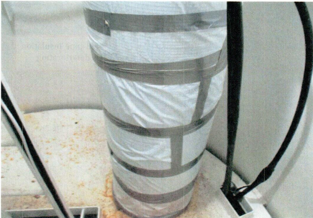
Top Platform - Good Condition - Minor Staining
