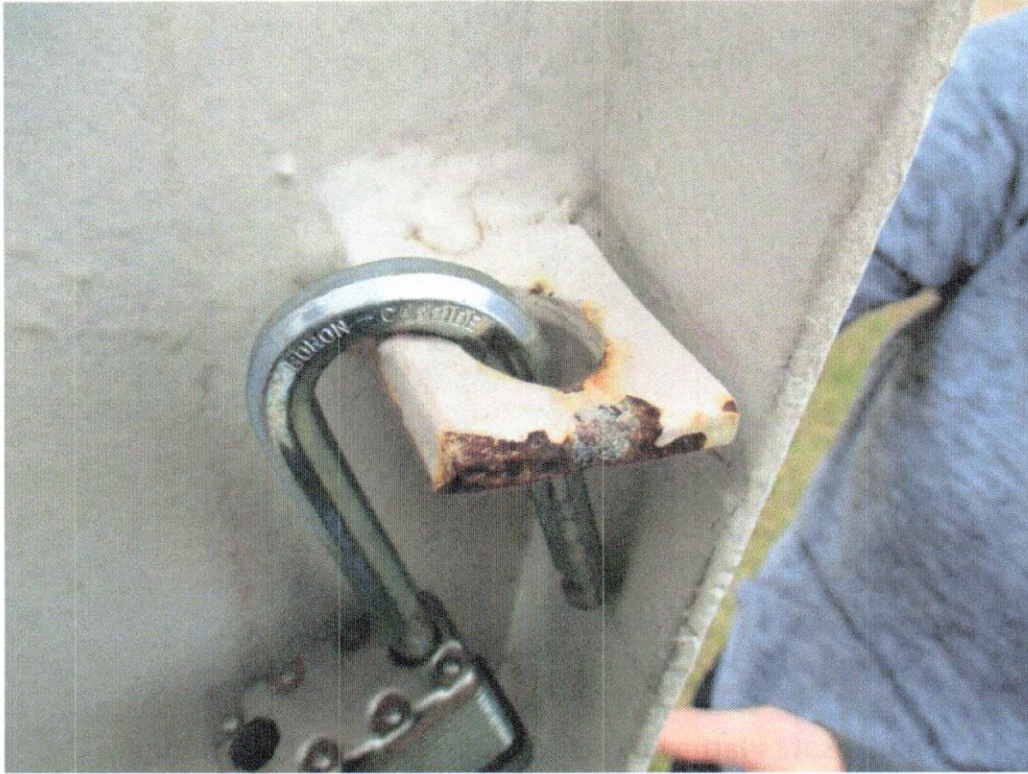
Tank Lock - Good Condition
