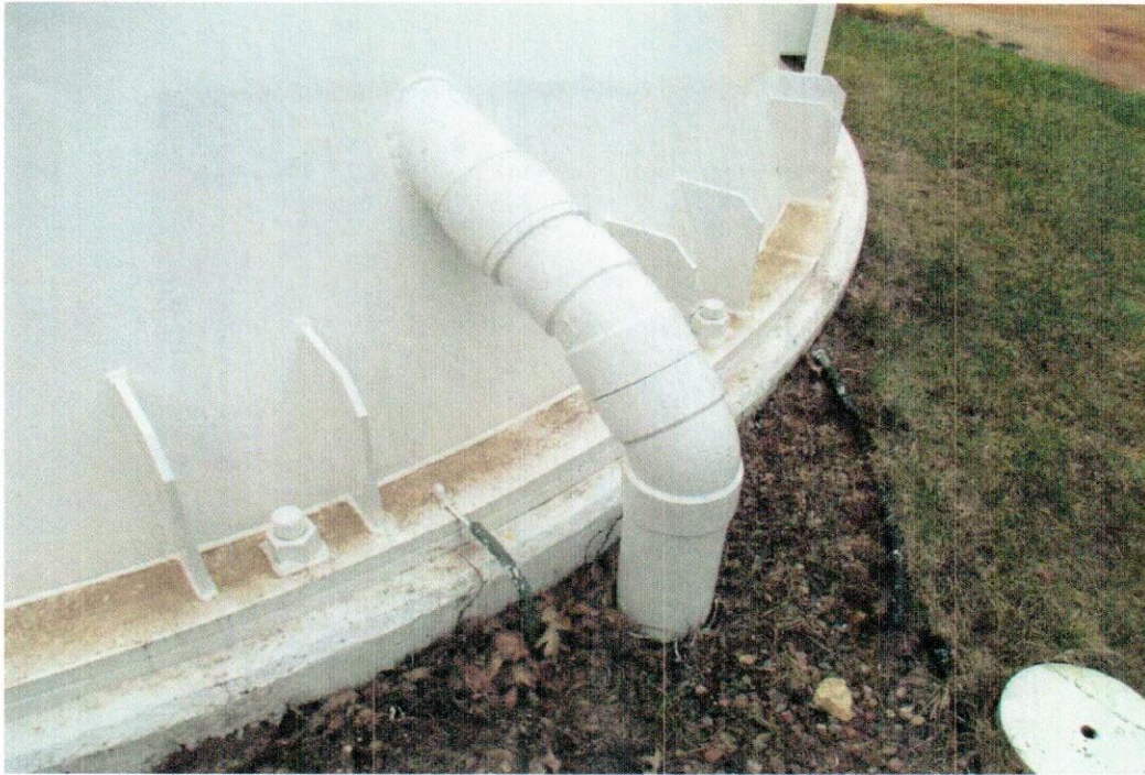
Exterior Foundation - Good Condition
