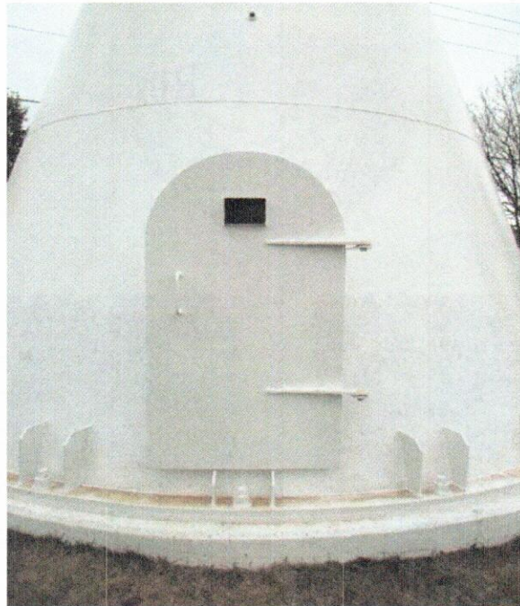
Exterior Door – Good Condition
