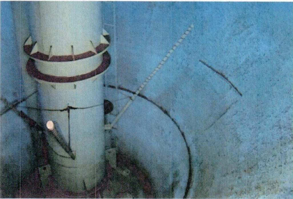
Interior Wet - Good Condition - Minor Sediment
