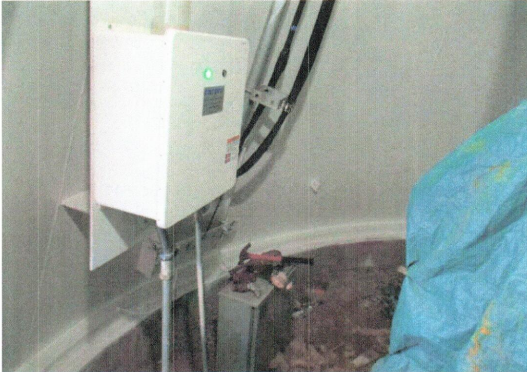
Interior Dry Base Bell - Good Condition
