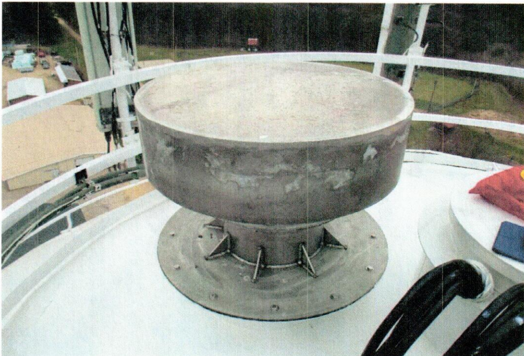
Exterior Roof Vent - Good Condition
