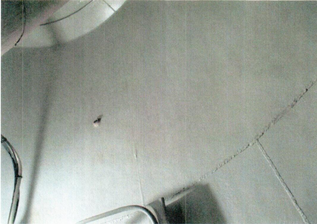
Interior Dry Base Bell - Good Condition
