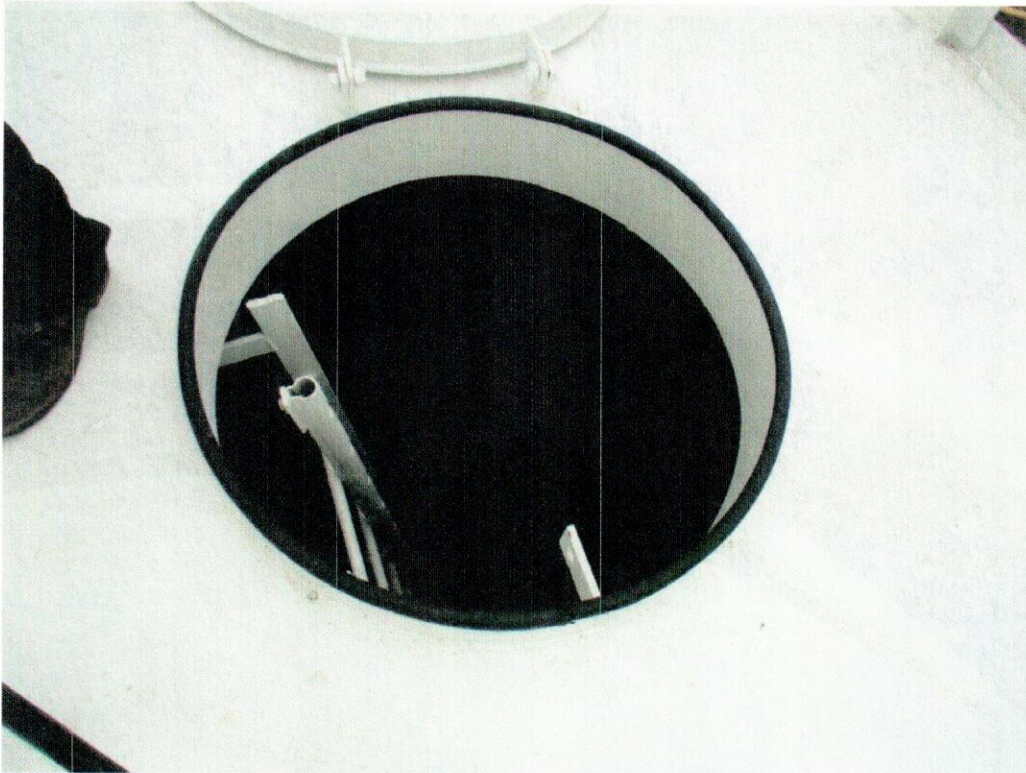
Exterior Wet Hatch - Good Condition
