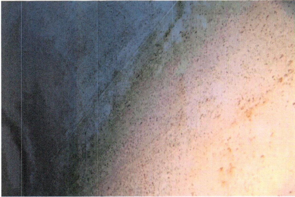
Interior Wet Sidewalls – Good Condition – Minor Staining
