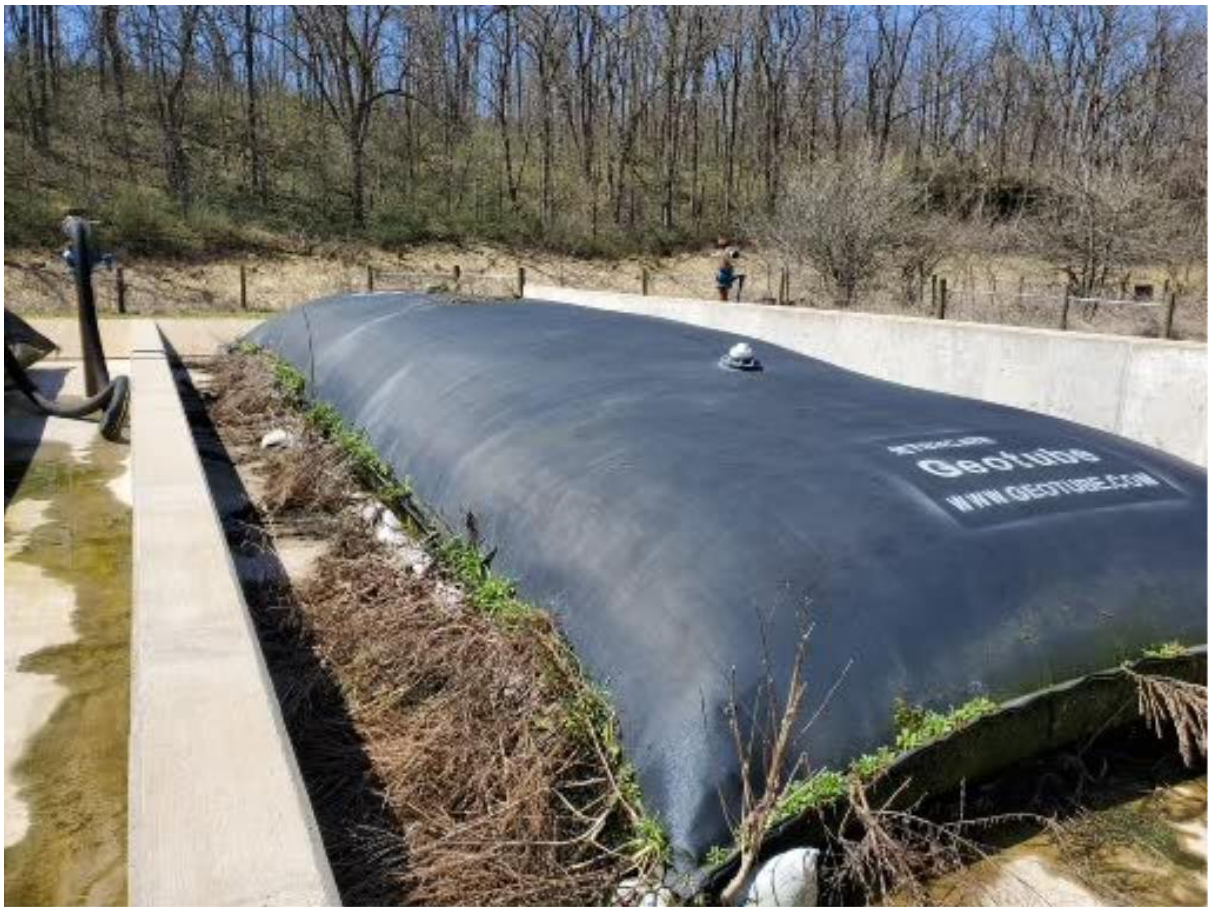
Picture #5 - Geotube Ready for Removal
