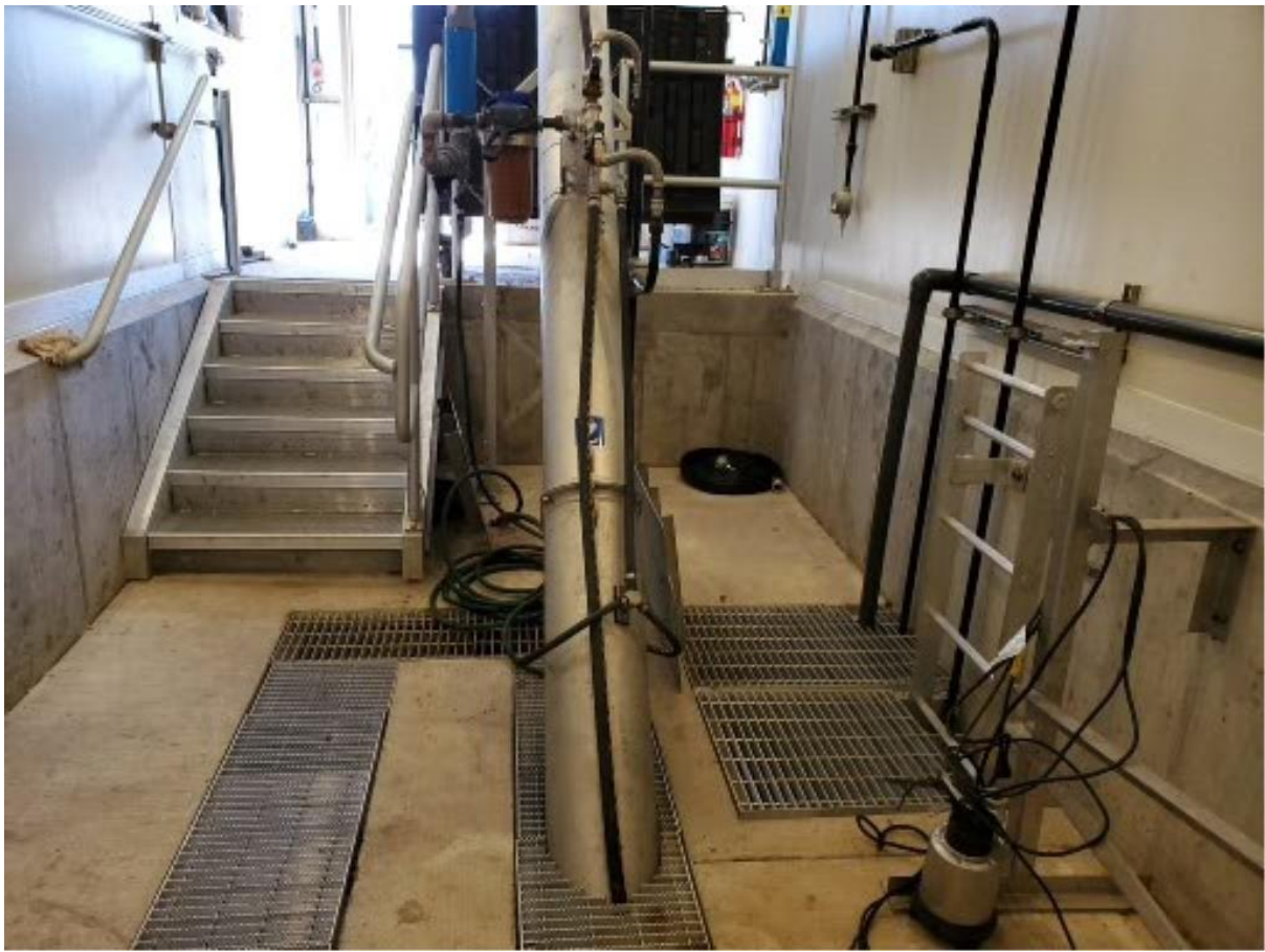
Picture #1 - Rotary Fine Screen at Headworks
