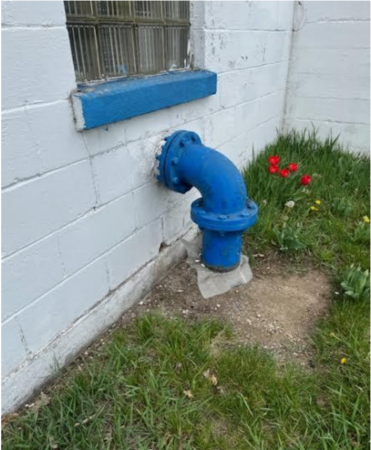
Overflow Pipe is in Good Condition
