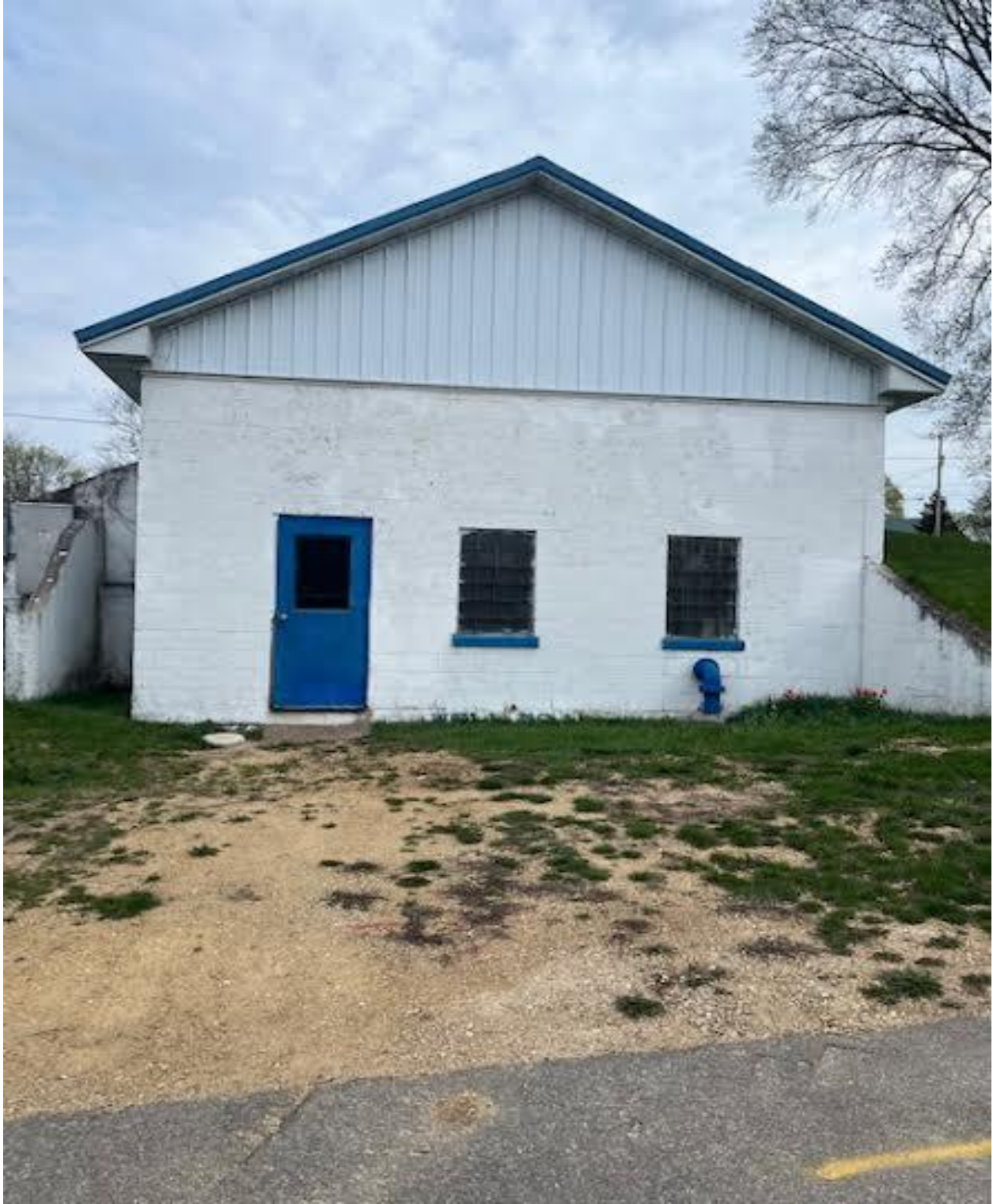
Well No #1 - 40,000 Gallon Concrete Reservoir
