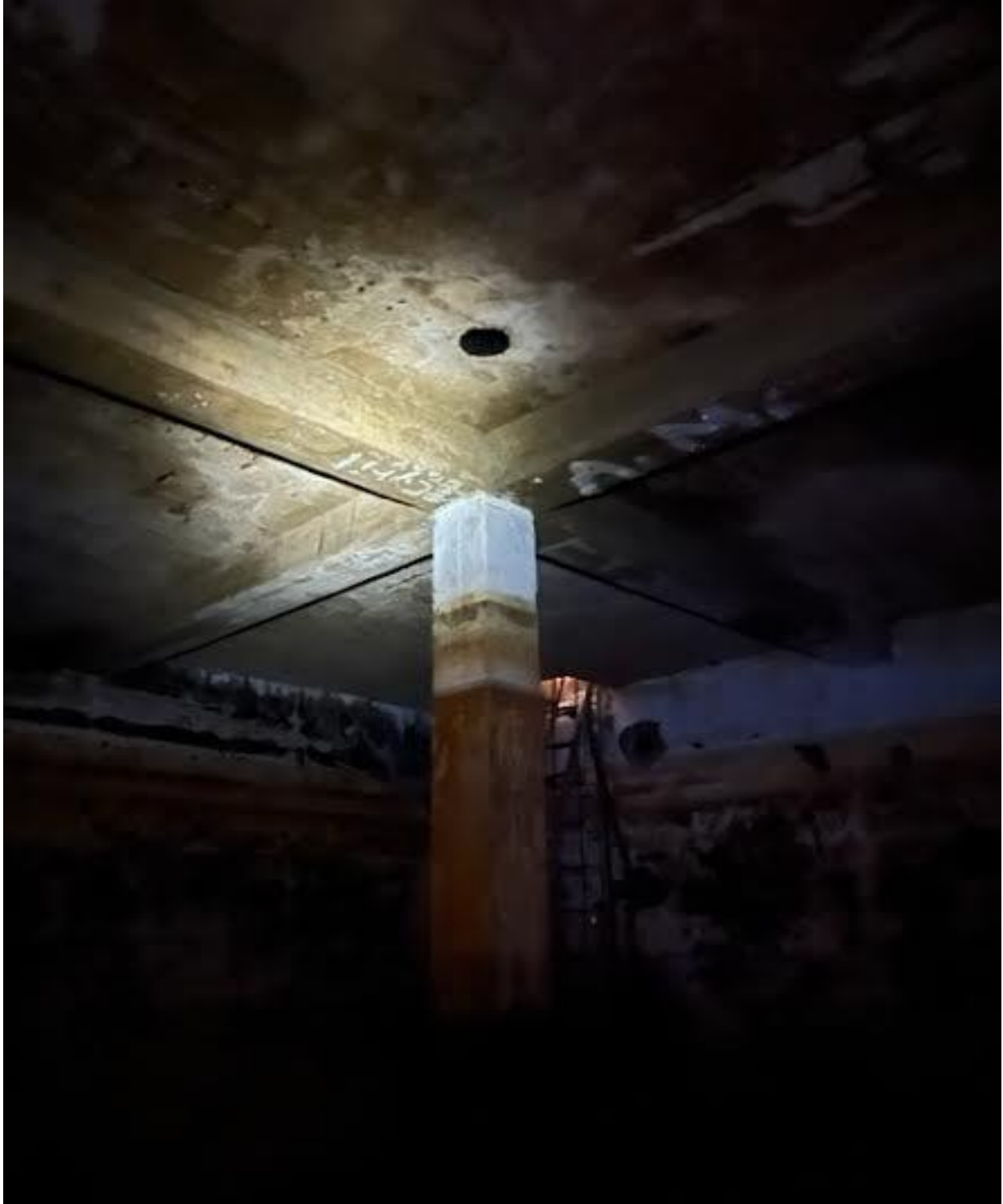
The Concrete Ceiling and Roof Vent Opening are in Good Condition
