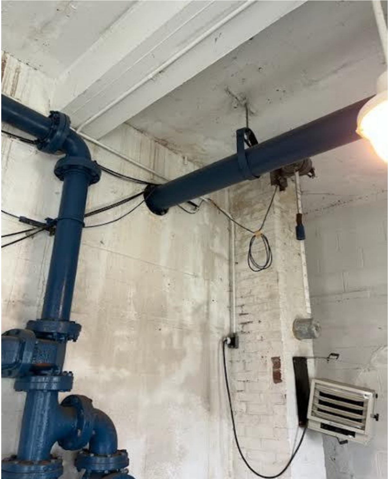
Overflow Pipe is in Good Condition
