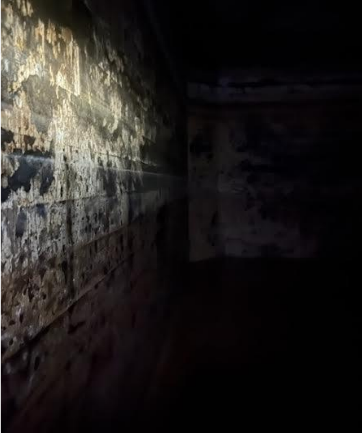
The Concrete Walls are in Good Condition
