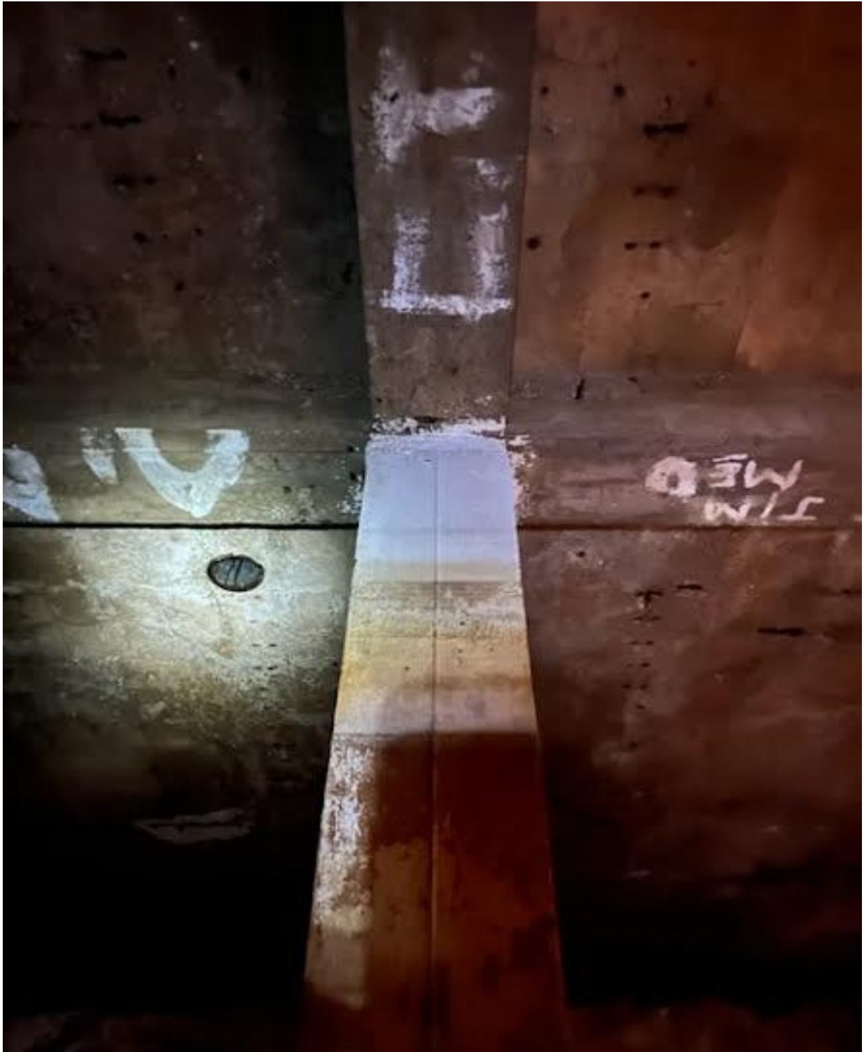
The Concrete Beams are in Good Condition
