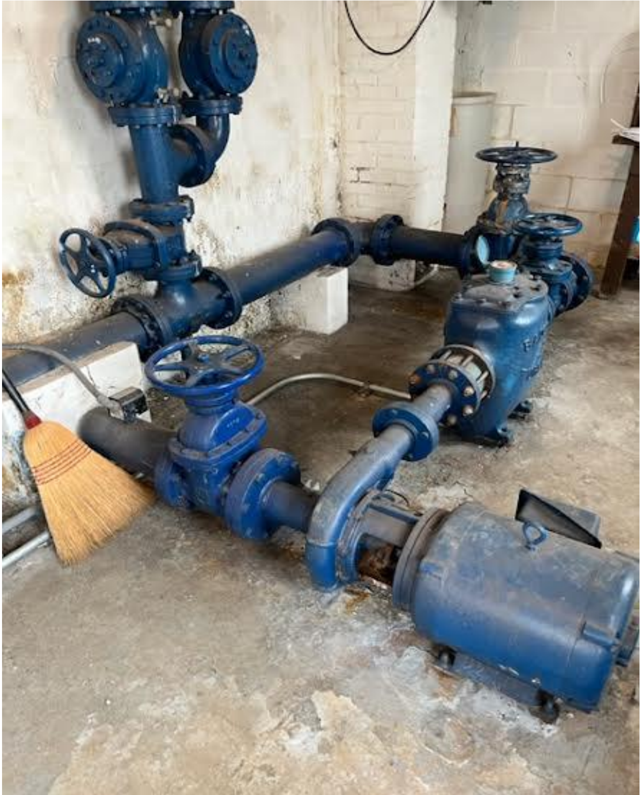
The Outlet Pipe is in Good Condition
