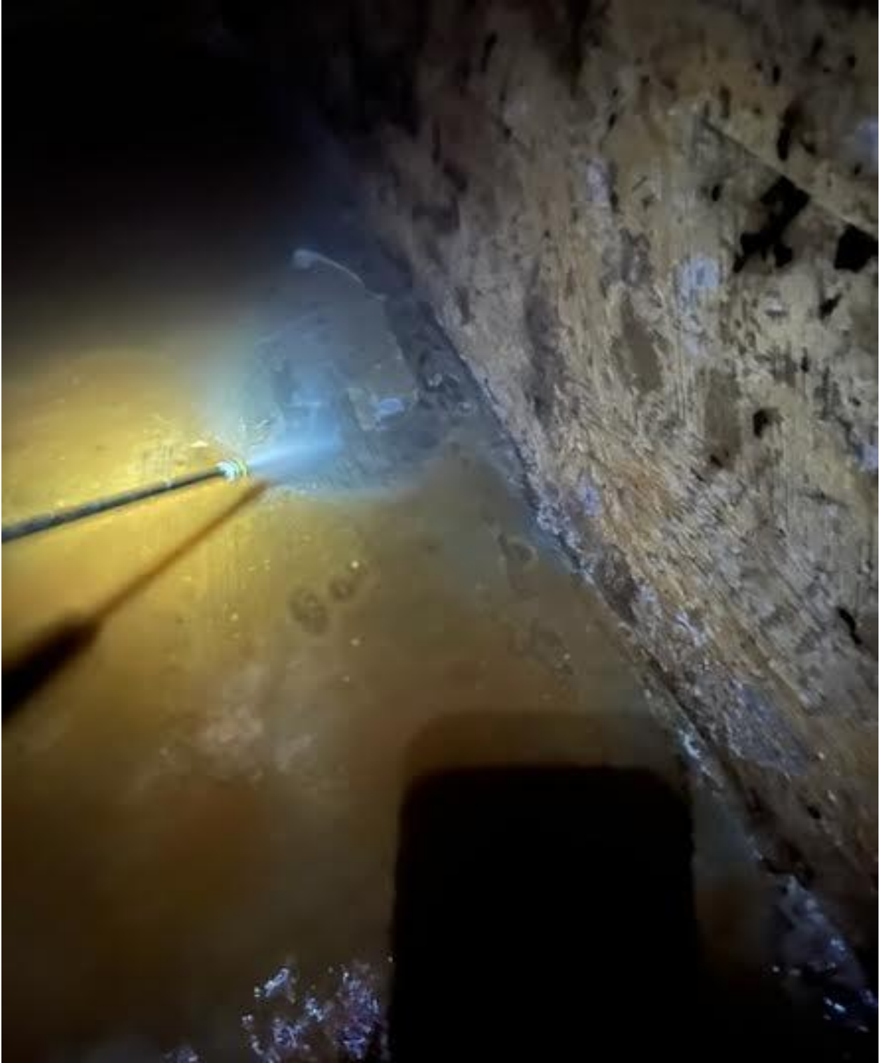
The Concrete Walls and Floor was Power Washed
