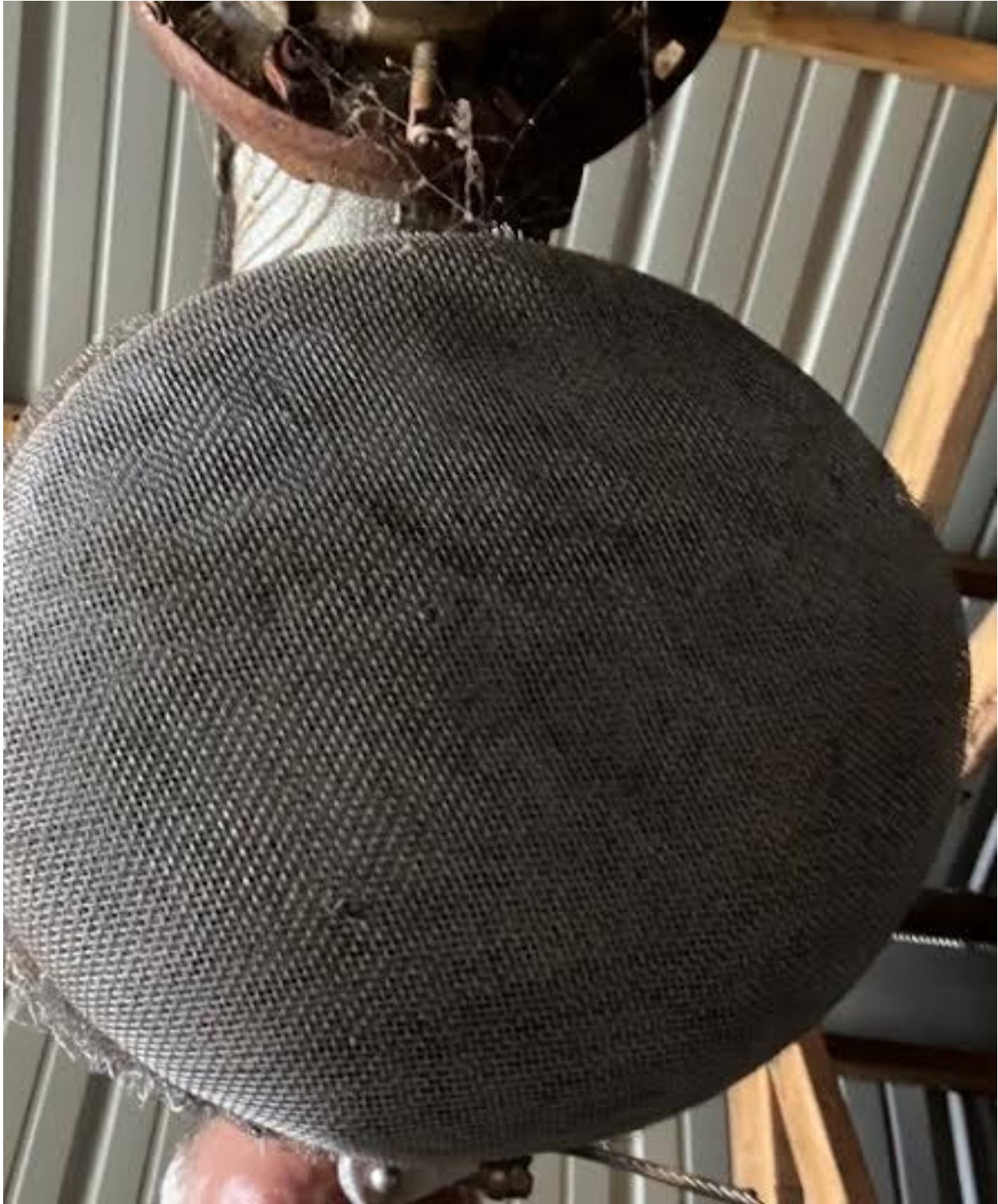
Vent Screen is in Good Condition
