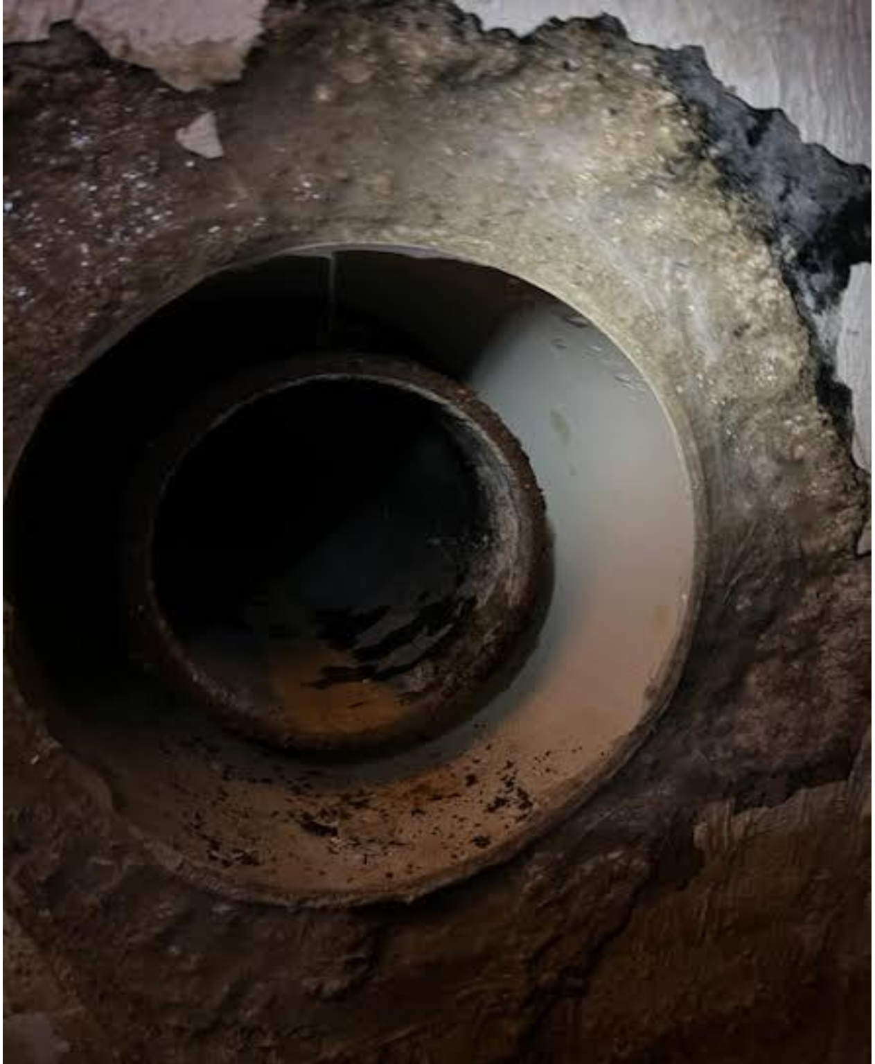
The Overflow Opening is in Good Condition
