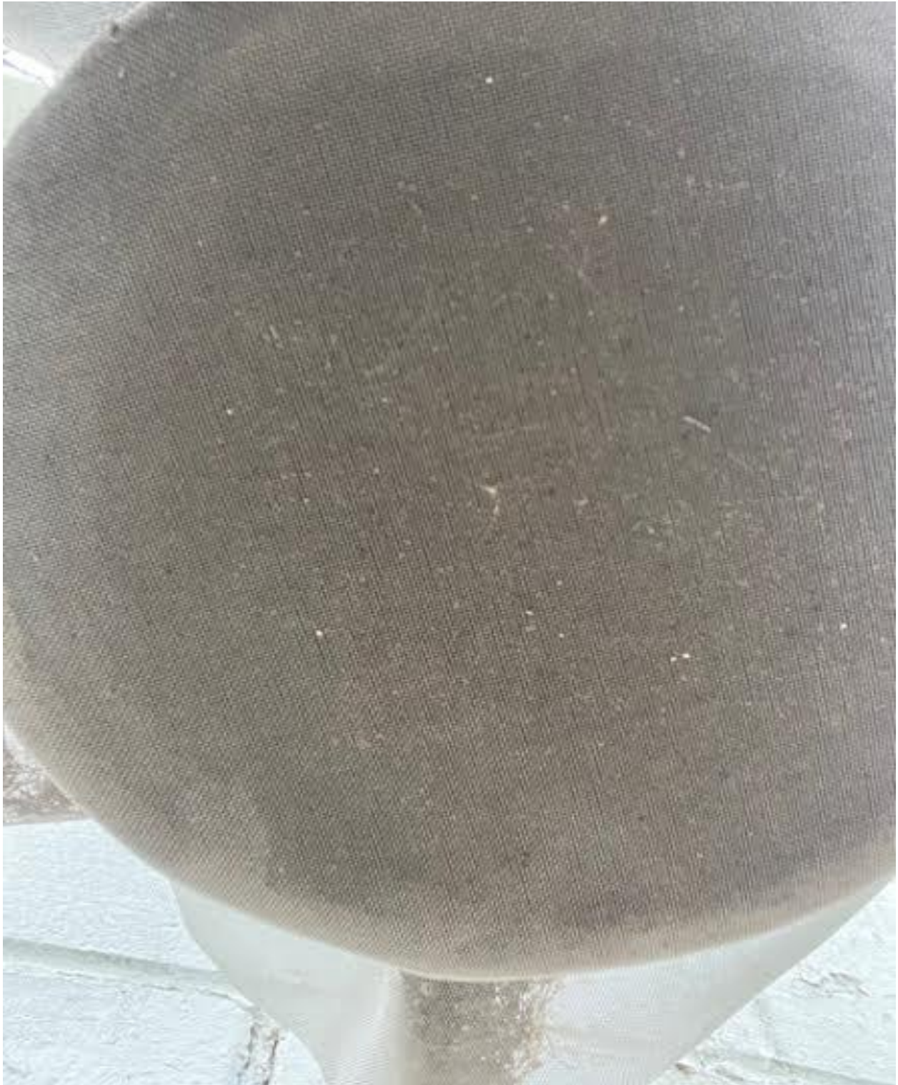
Overflow Screen is in Good Condition
