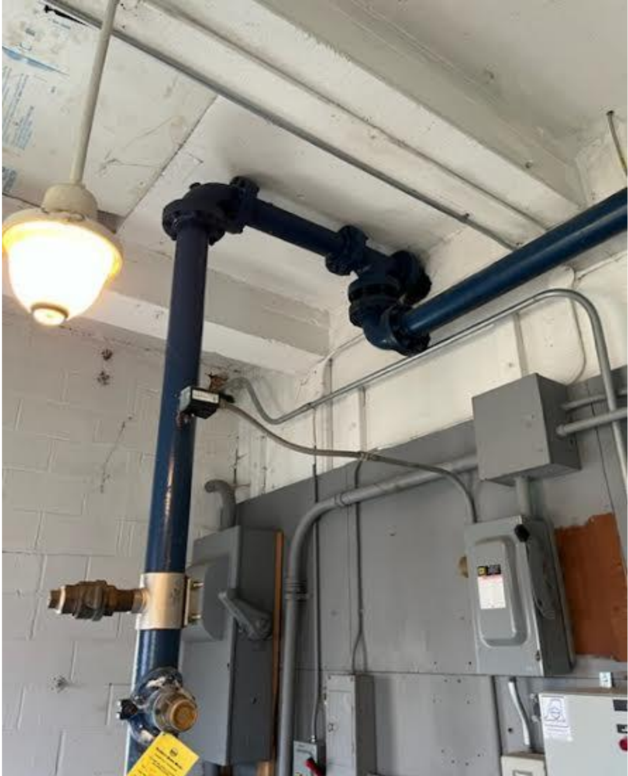
The Fill Pipe is in Good Condition
