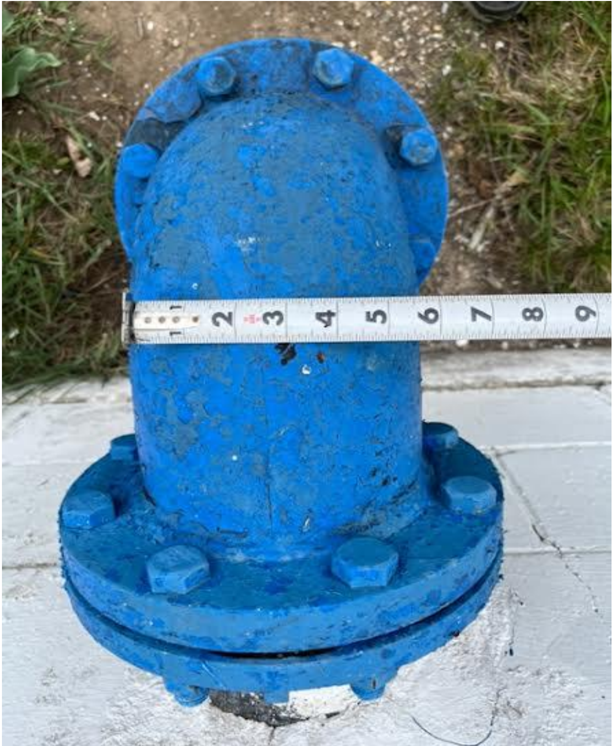
6" Overflow Pipe is in Good Condition
