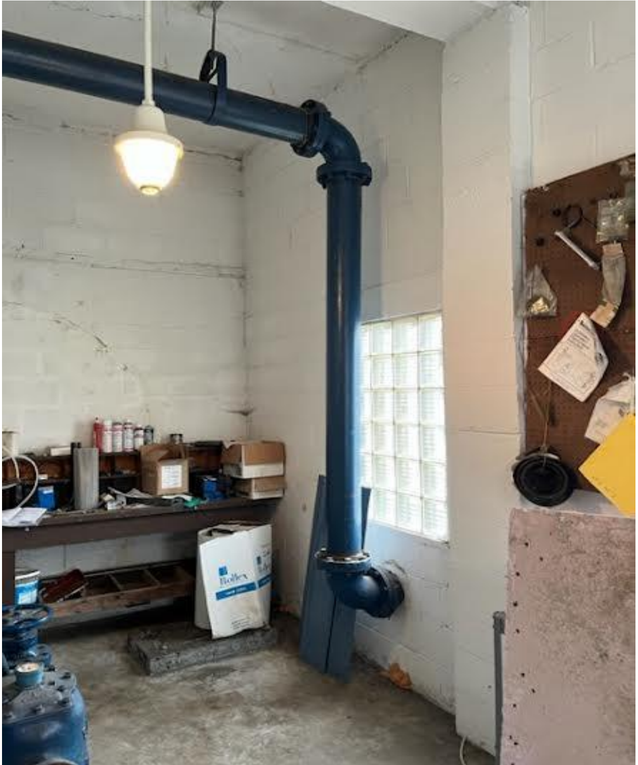
Overflow Pipe is in Good Condition
