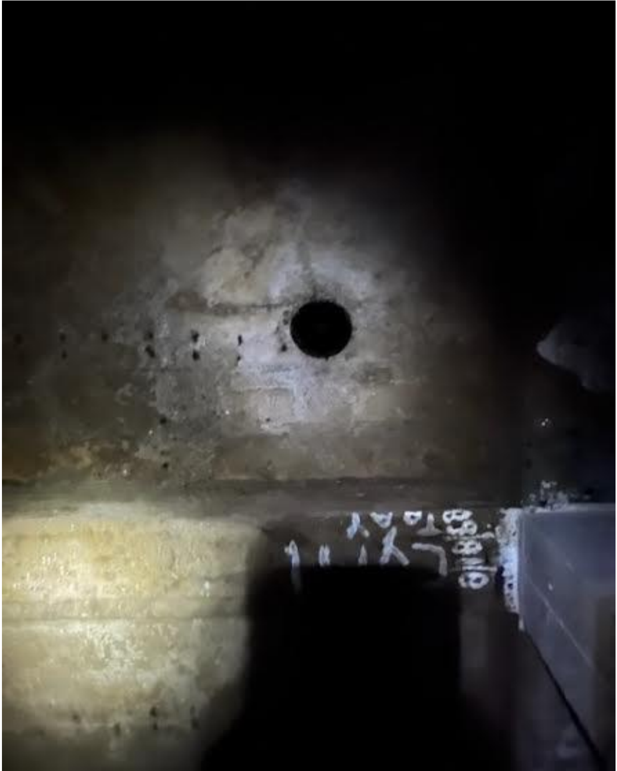
The Roof Vent Opening is in Good Condition
